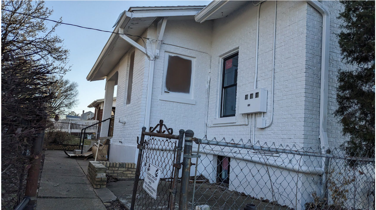
East Rear Façade
