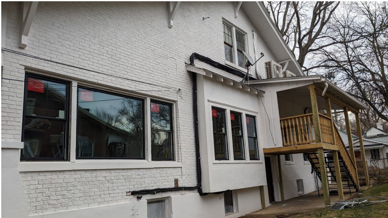
South Side Facade
