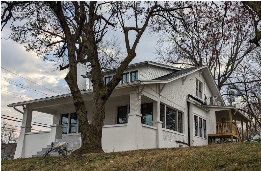
Front (west) and Side (south) Façades
