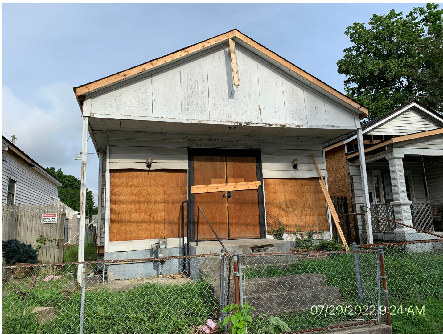
Left of subject property.
