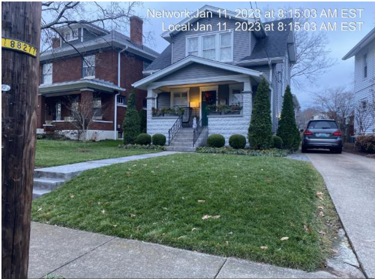
Front of subject property.
