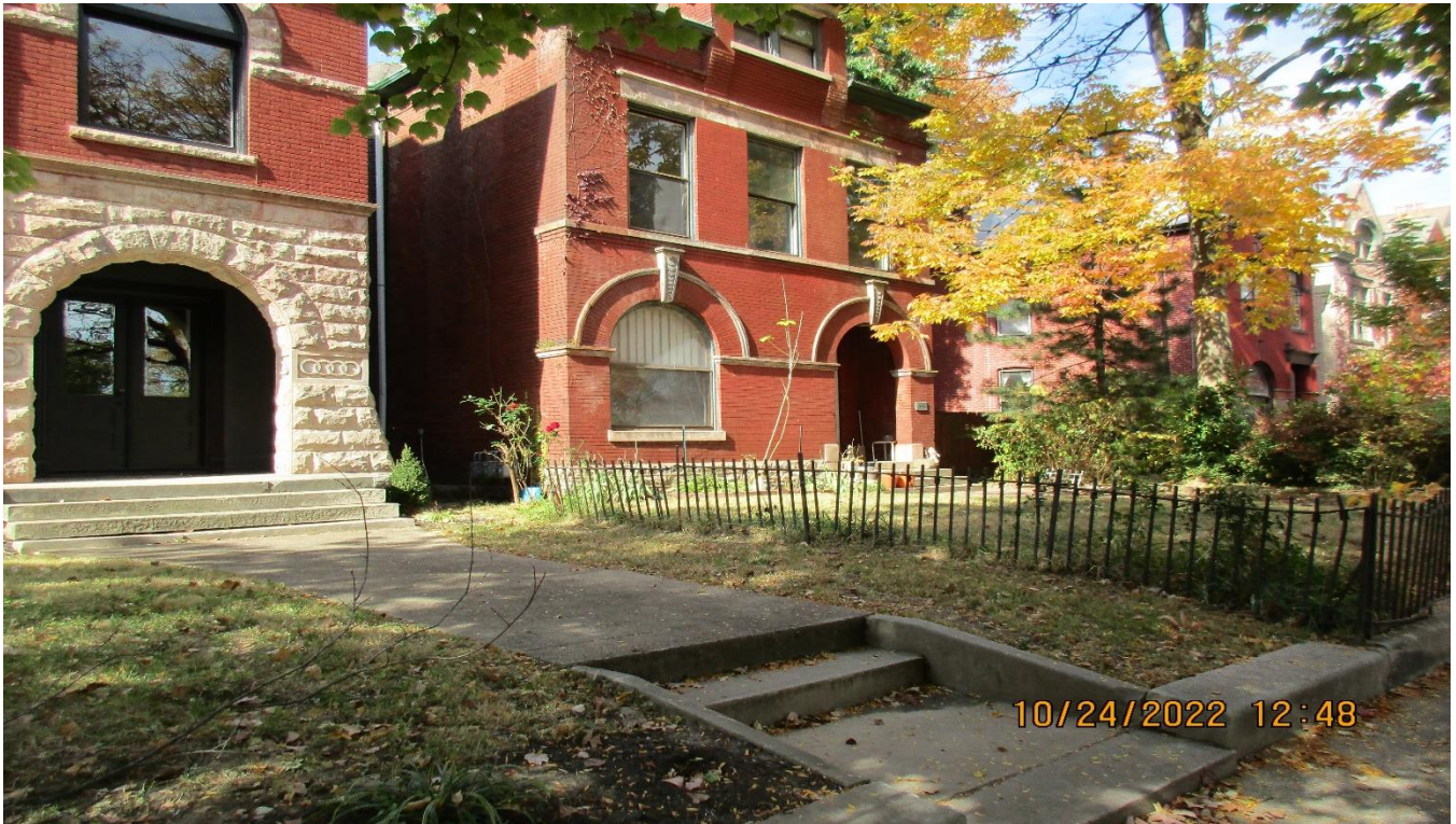
Property to the right of subject property
