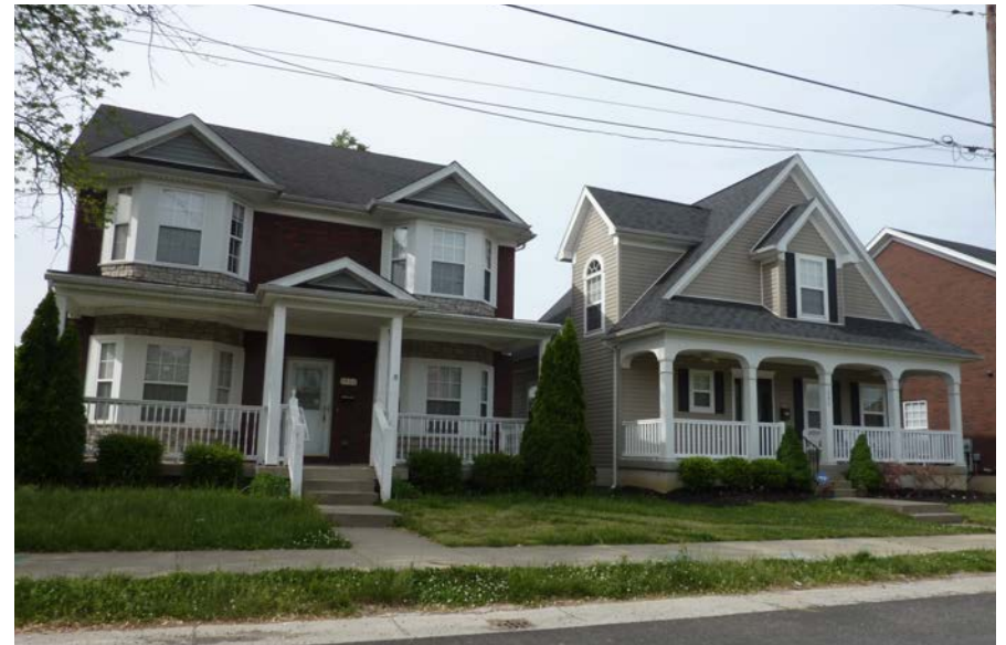
Recent housing construction in Russell
