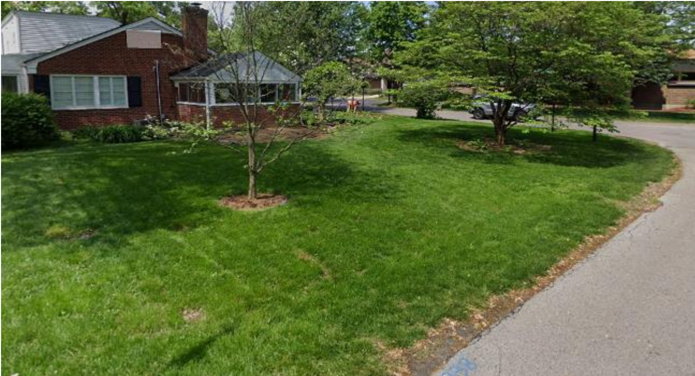
View of subject property at corner of Brookfield Avenue and Cherrywood Lane
