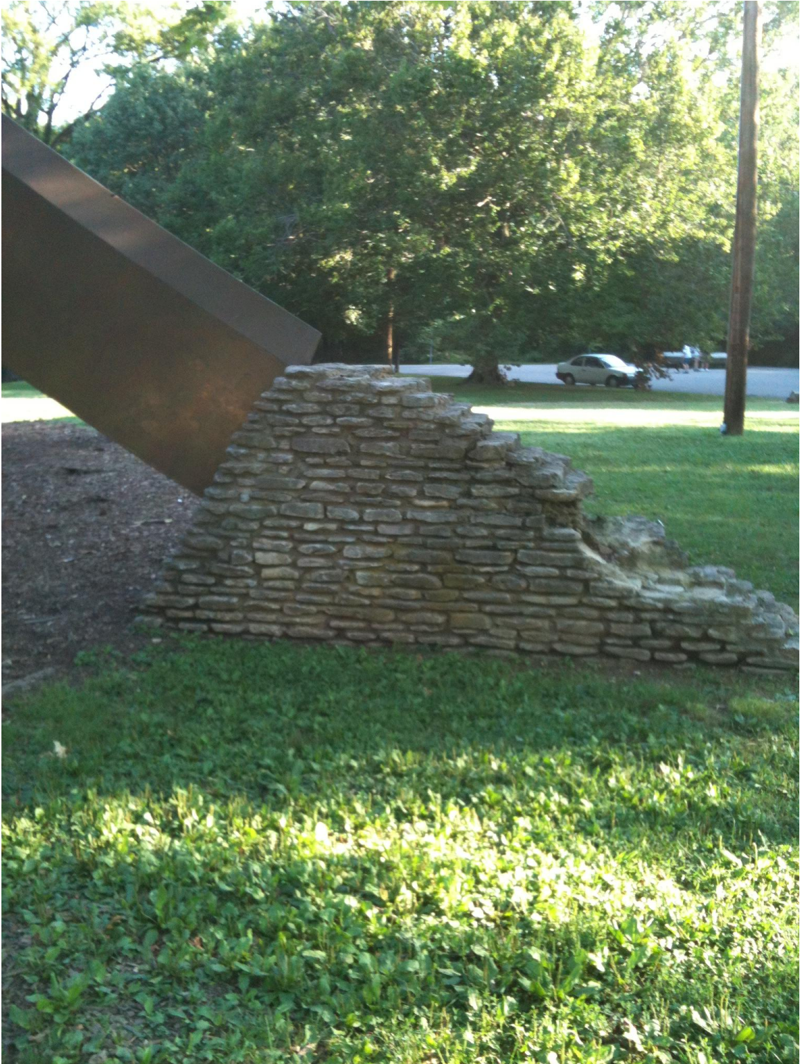
Detail of buttress element
