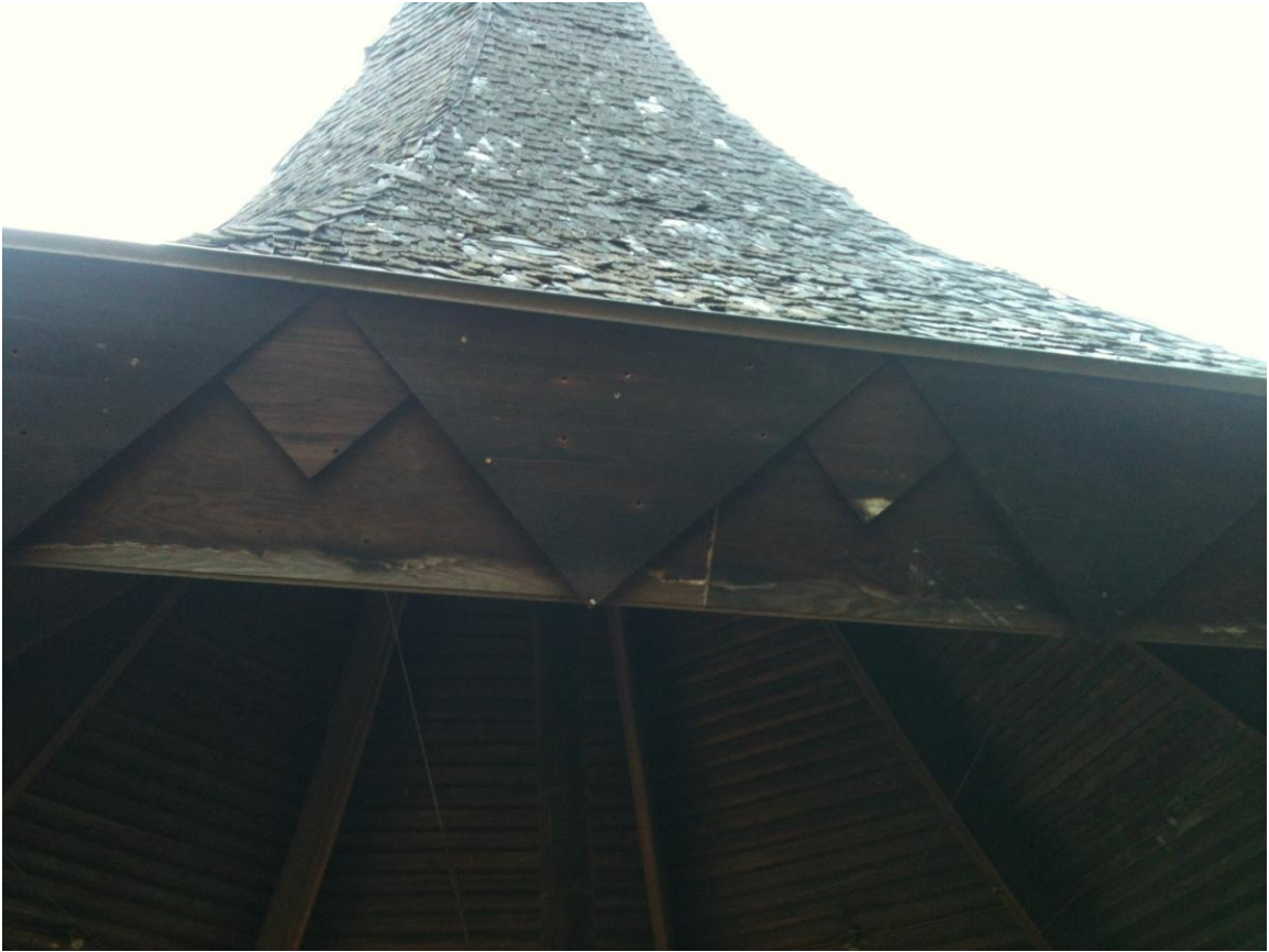
Detail of fascia board dentil pattern
