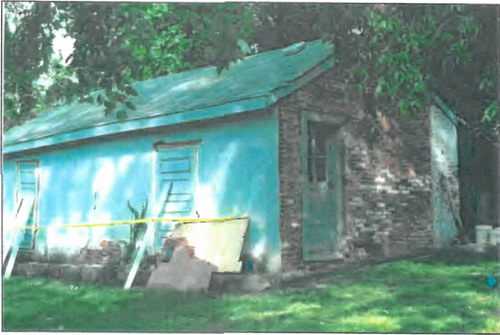
Figure 7. Photograph of Slave House (North and West Sides).
