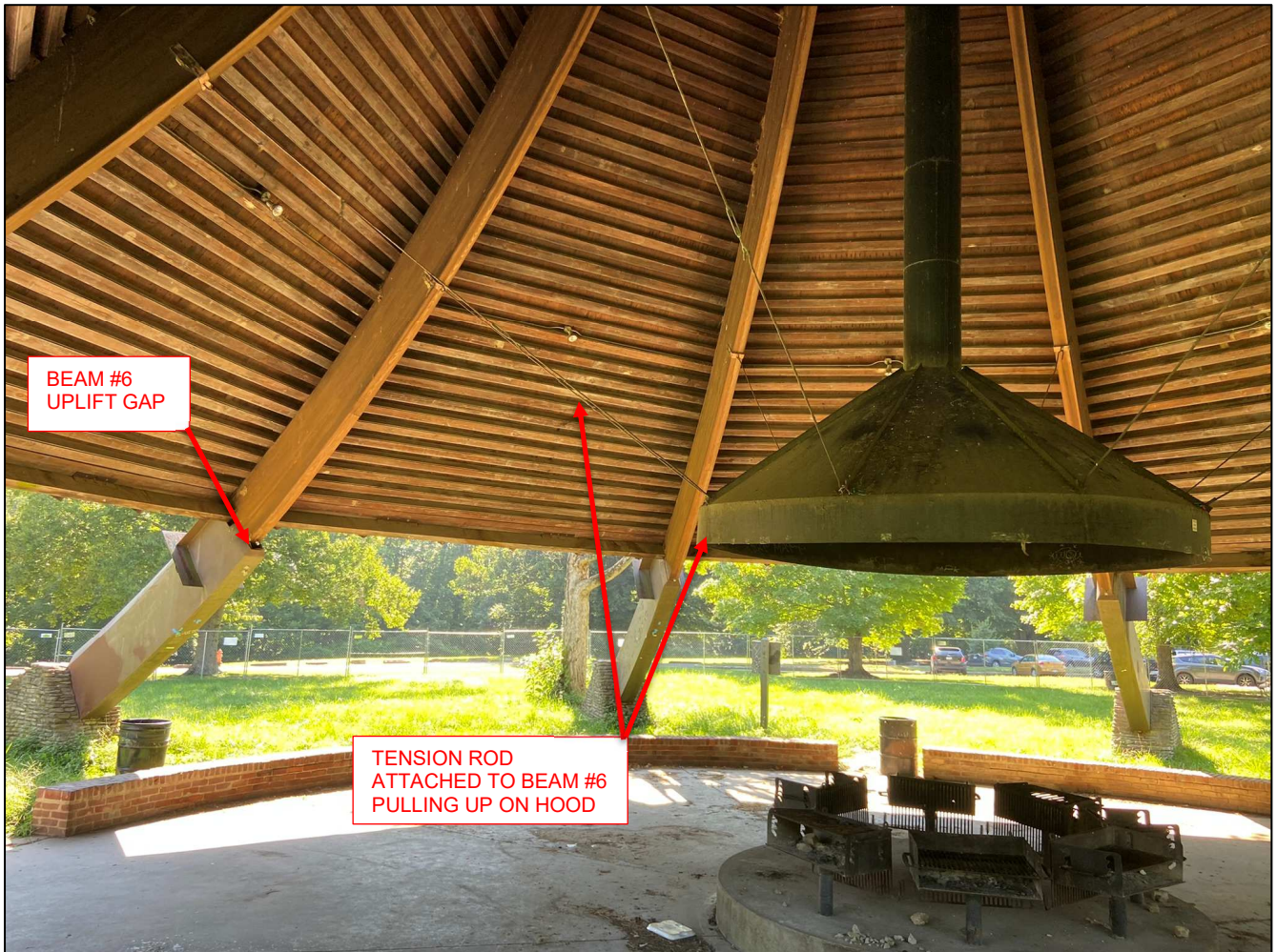
Photo 5: Hood Lifting from Beam #6 Movement
