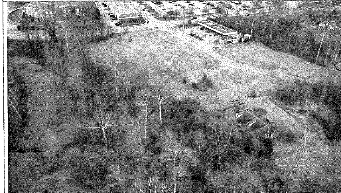
Photo 2. Site Looking Northeast Toward Slope at West Perimeter of Proposed Pavement
