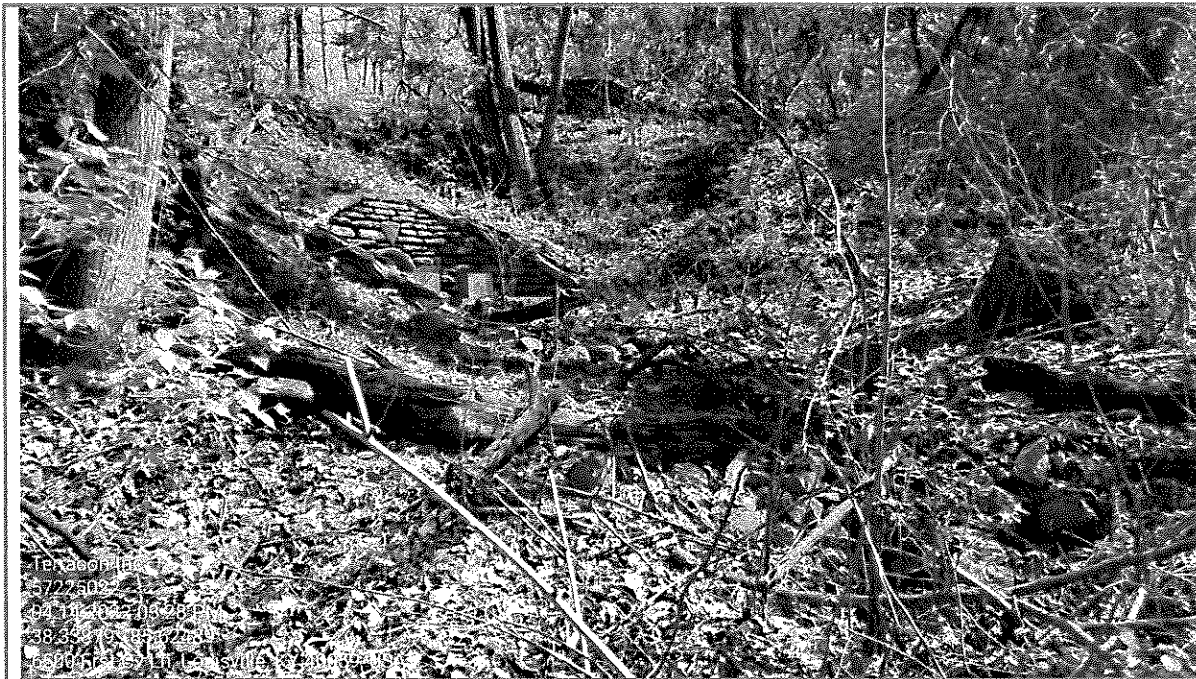
Photo 7. Site Looking Southeast Toward Culvert Headwall Structure at West
