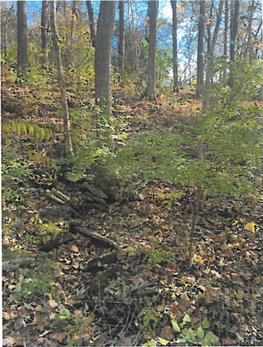
Area 8: Rock Outcropping, Minor Instability
