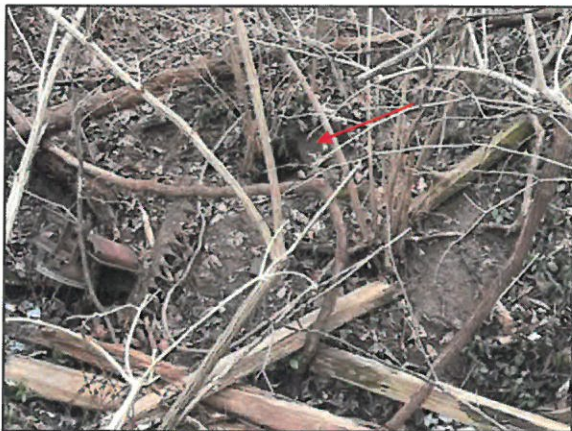
PHOTO NO. 10: Conduit/ swallow hole at Feature 7
