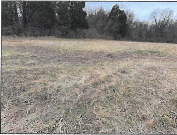
PHOTO NO. 6: Ground subsidence (Features 5 and 6)
