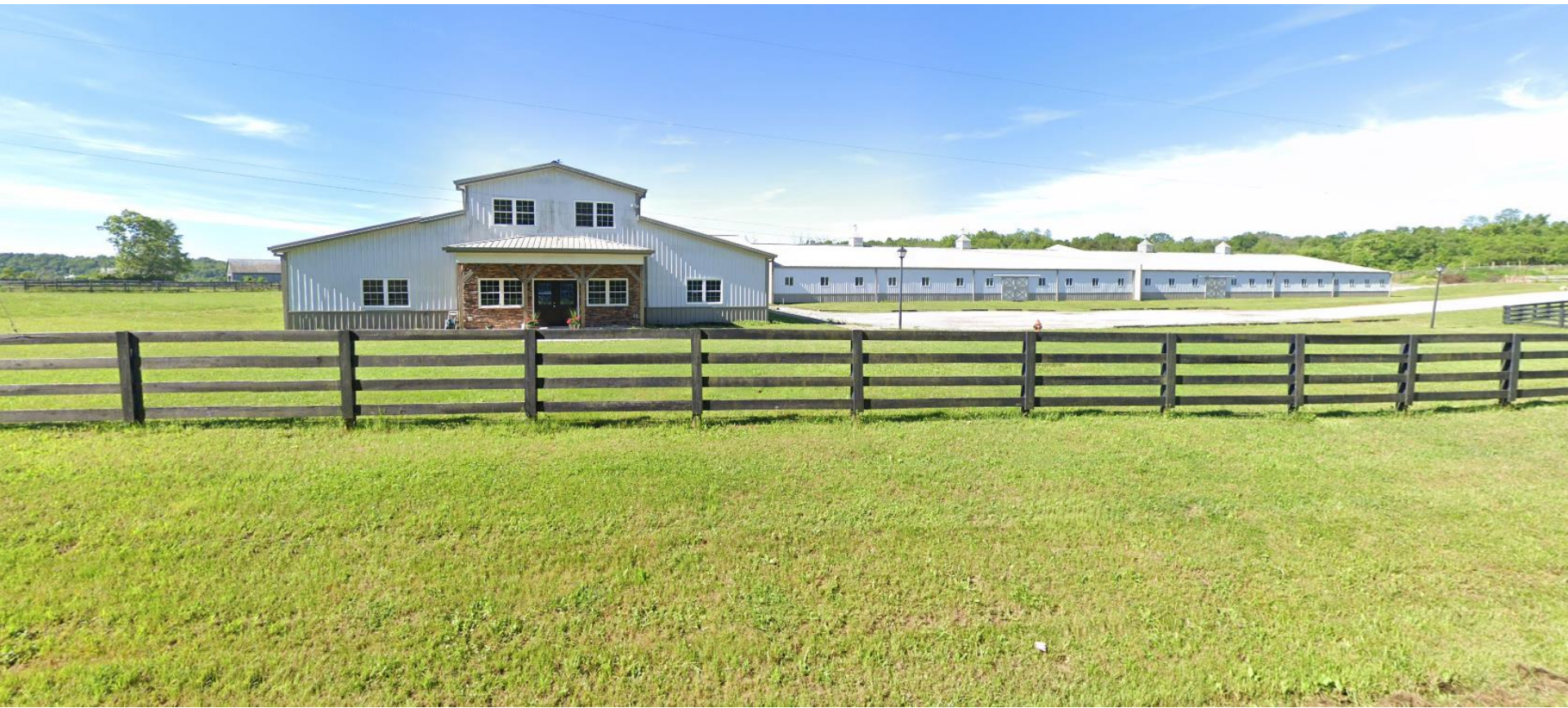
View of existing buildings to remain.
