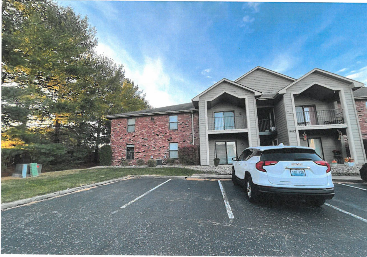
Example of 2-story building turned perpendicular to abutting property with berm, privacy fence, and tree combo. (Hurstbourne Crossing - Hurstbourne Pkwy)
