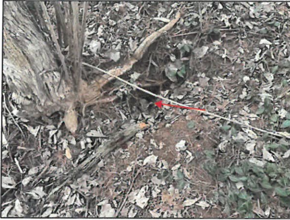
PHOTO NO. 5: Sinkhole conduit/throat (Feature 4)
