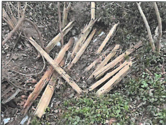
PHOTO NO. 9: Sinkhole at southwest corner (Feature 7)
