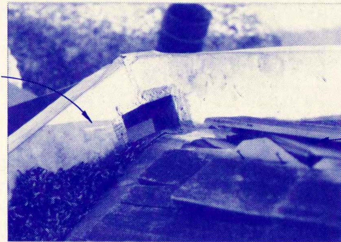
REMOVE EXISTING COPPER GUTTER LINER AND REPLACE AS DETAILED ON SHEET S-2
