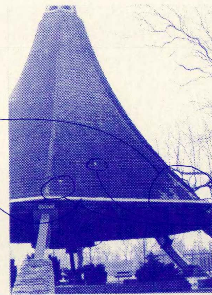
ROOF SECTION NO. 7
