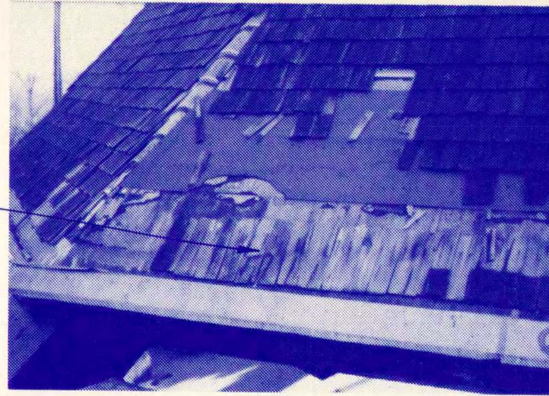
REMOVE ALL NAILS AND ASPHALT SHINGLES WHERE SHAKES AND GUTTER LINER ARE TO BE INSTALLED
