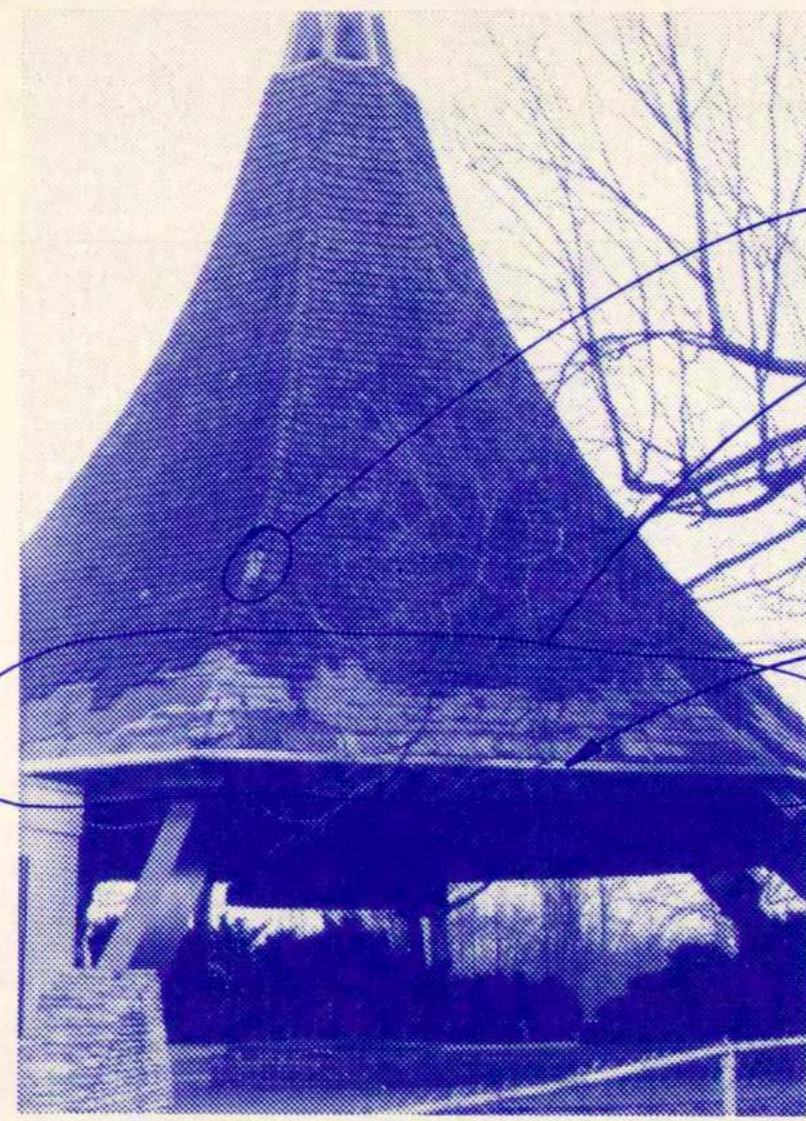
ROOF SECTION NO. 1
