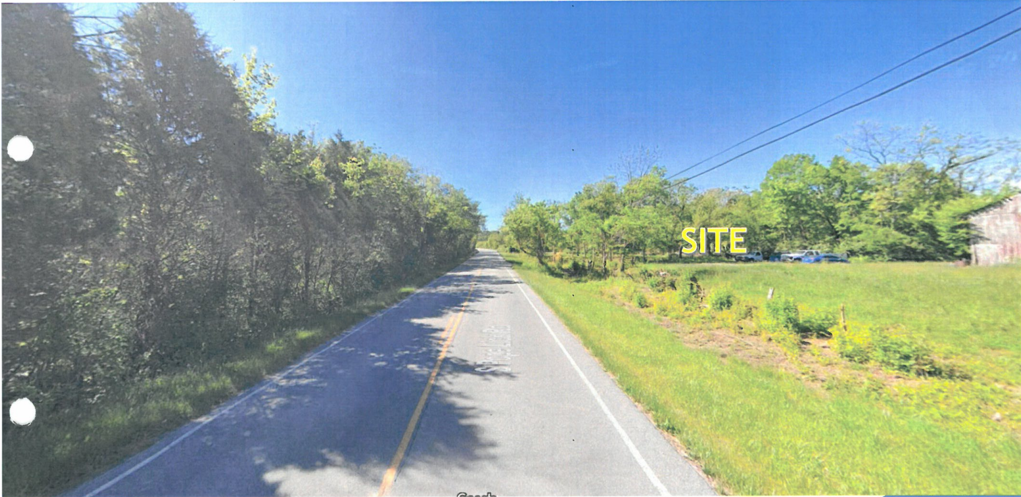
View of S. Pope Lick Road looking south. Site is to the right.
