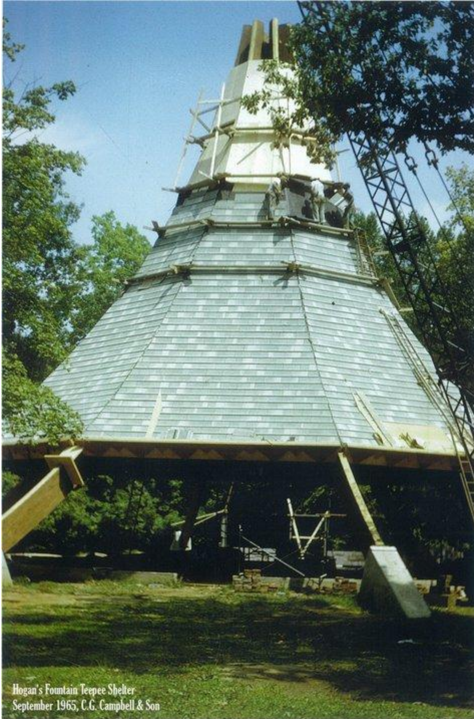
September 1965, Shelter under construction
