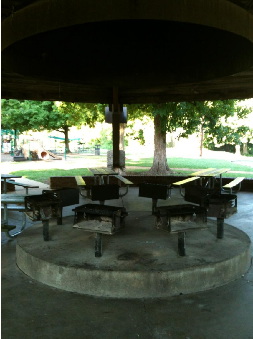
Location of fire pit (removed) with grills in place currently
