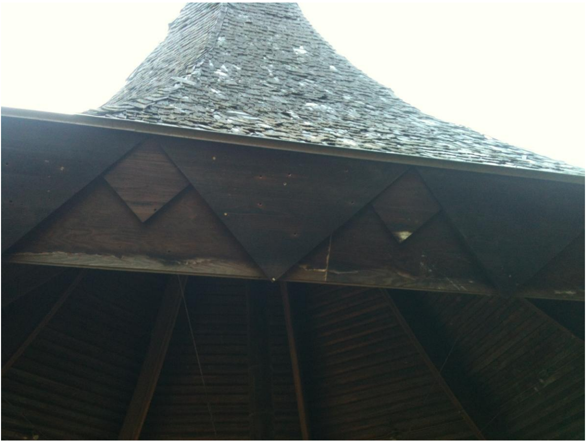
Detail of fascia board dentil pattern
