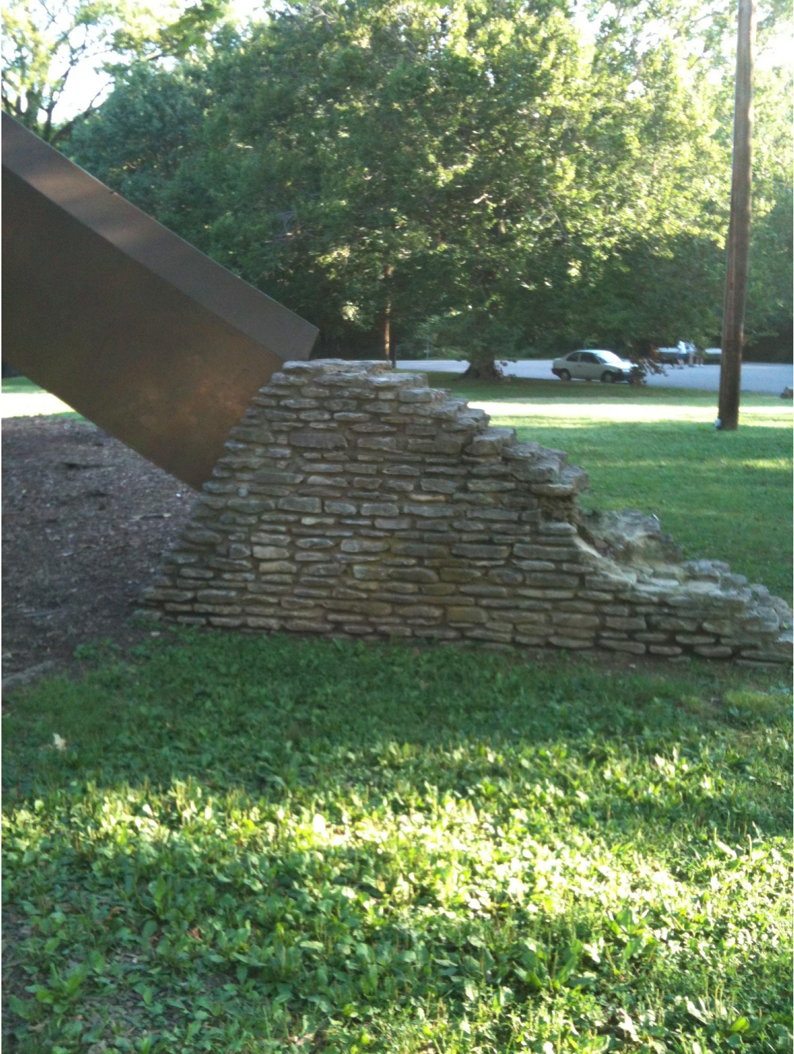
Detail of buttress element
