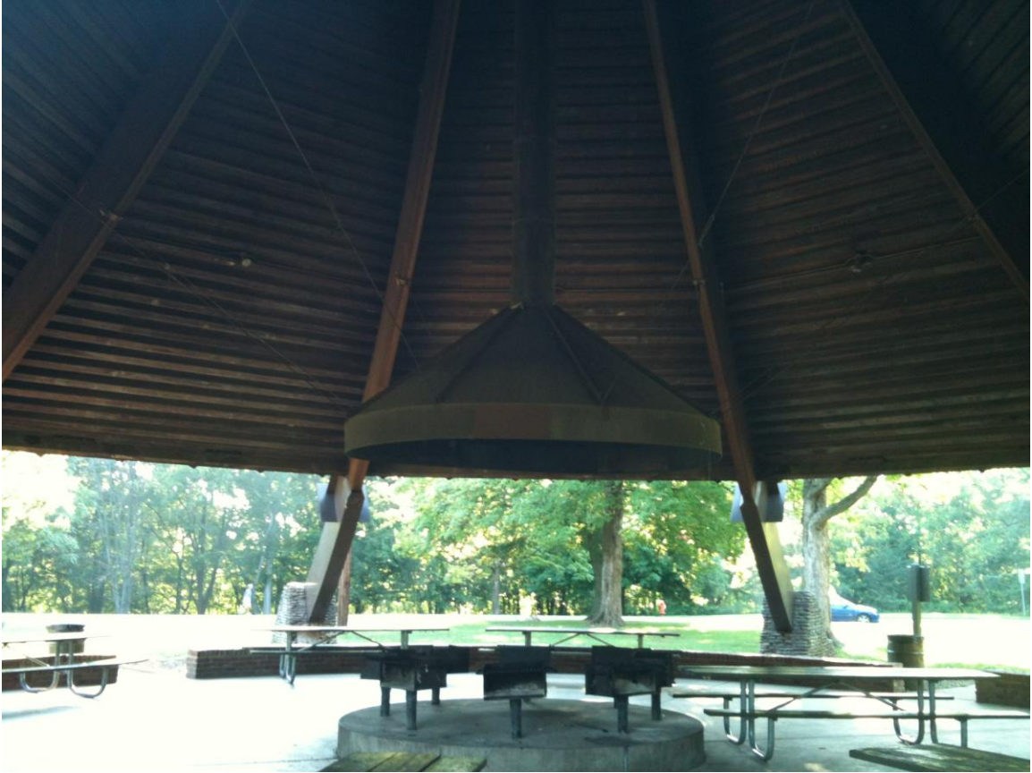
Interior of shelter
