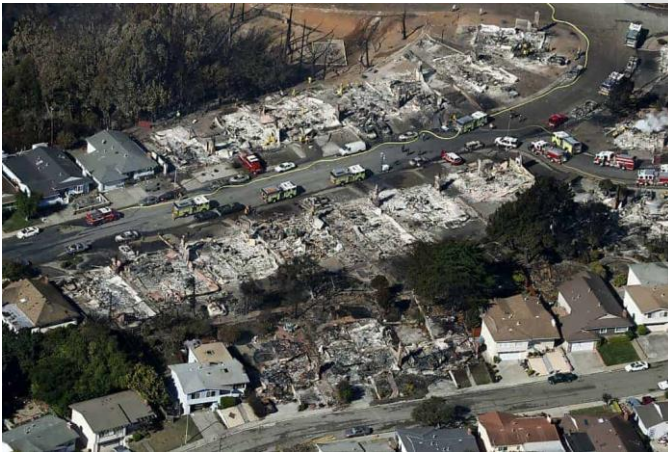
Hill Street after the 1981 Sewer explosions Source: historycollection.com
