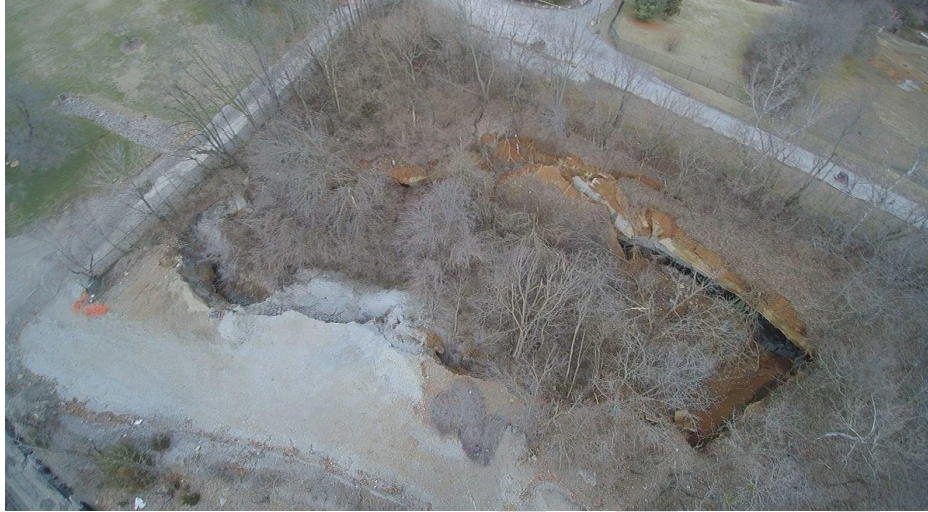
Louisville Zoo Sinkhole Photo: Wave3
