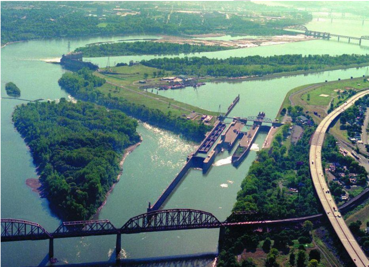
McAlpine Locks and Dam, Louisville, KY Source: U.S. Army Corps of Engineers
