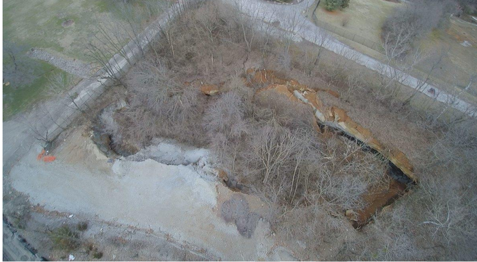
Louisville Zoo Sinkhole Photo: Wave3
