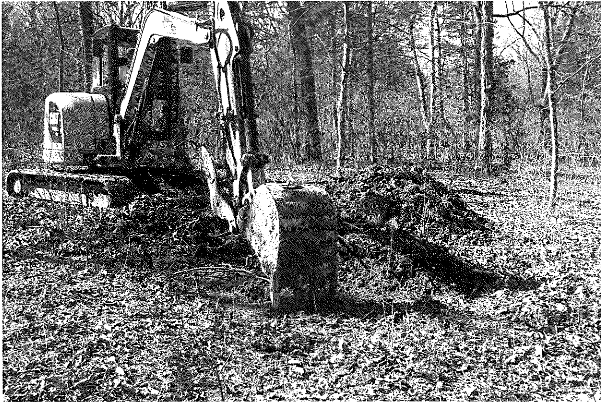
Figure 7. Excavation in progress at Cemetery 2.
