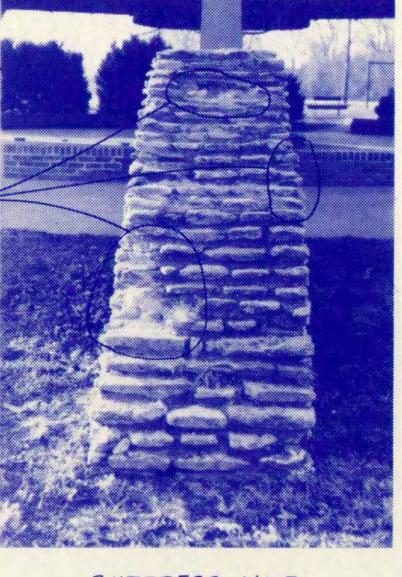
STONE BUTTRESS REPAIR (SEE SHEET S-I FOR SECTION LOCATIONS)
