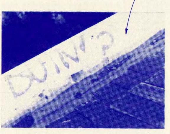
REMOVE ALL NAILS AND ASPHALT SHINGLES WHERE SHAKES AND GUTTER LINER ARE TO BE INSTALLED
