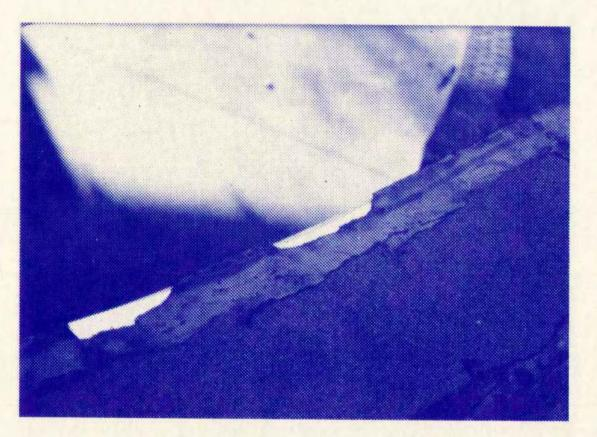
REPAIR BATHROOM BUILDING ROOF AS NECESSARY WITH ASPHALT ROOF COATING
