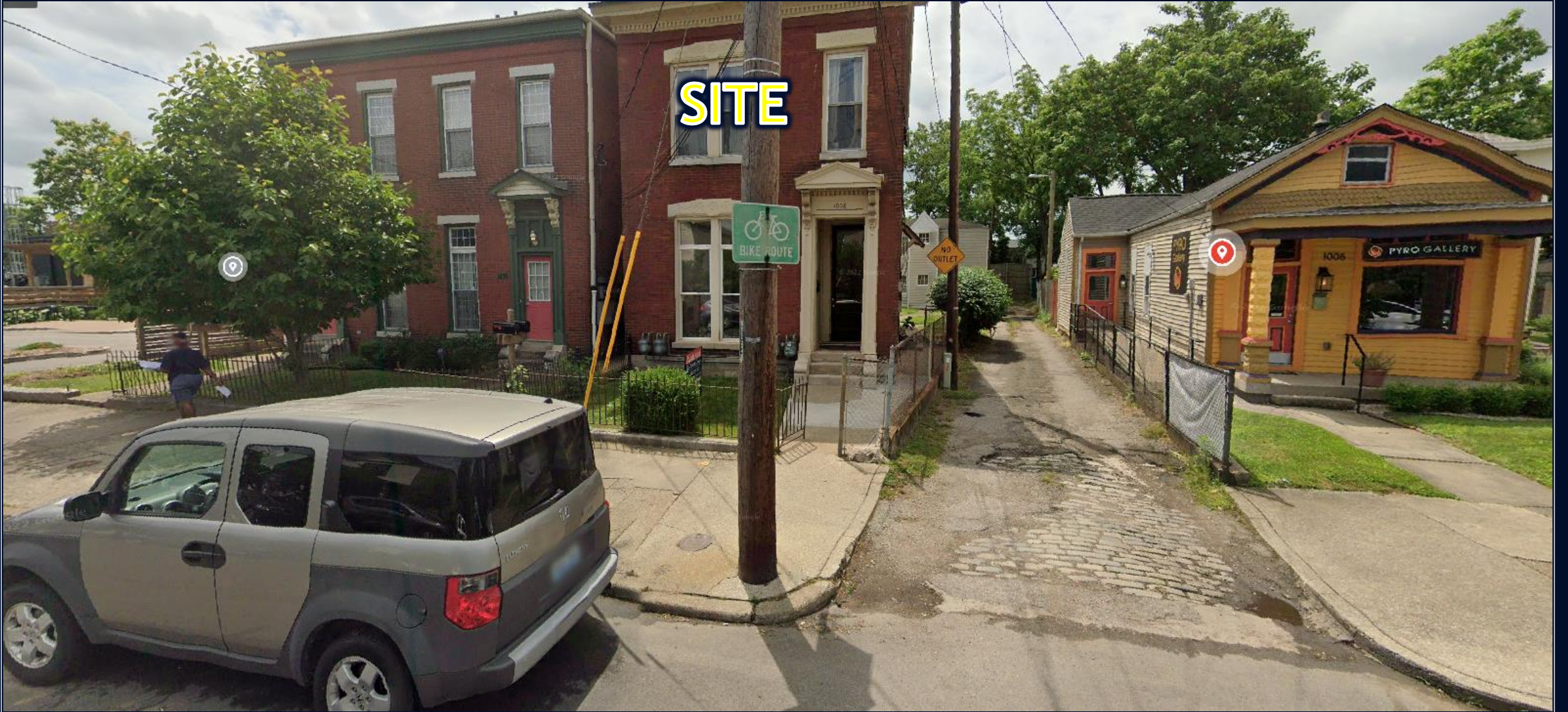
View of site from E. Washington Street.
