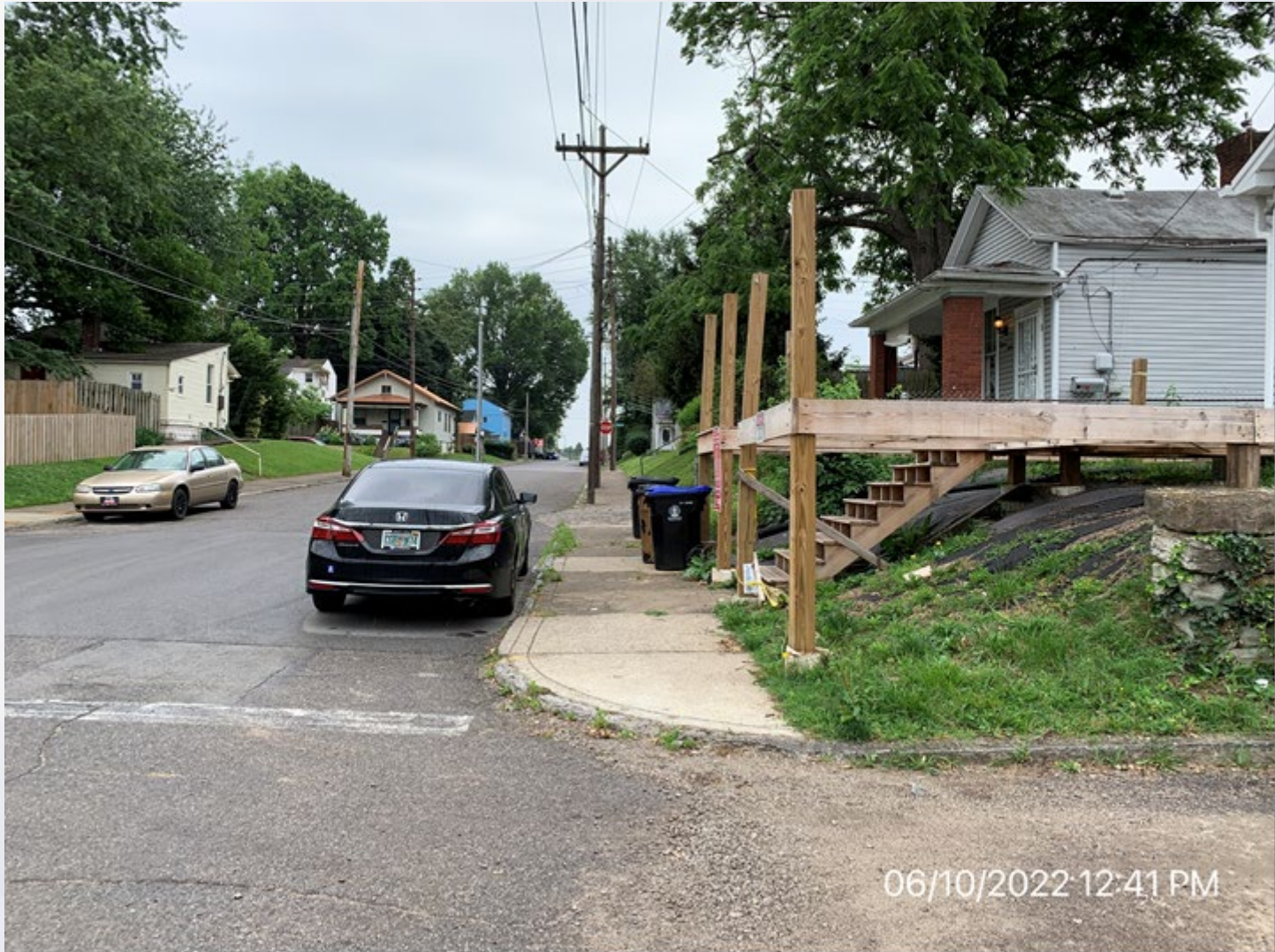
View of deck from intersection of alley and Hoertz Ave.
