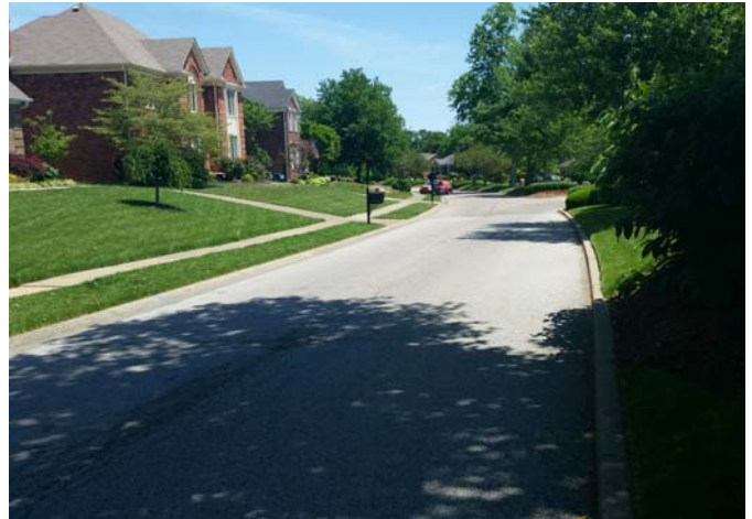
Photo #14: Southbound lane looking northeast near 506 Lake Forest Pkwy.
