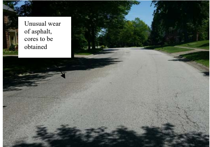
Photo #8: 2-way roadway section looking northeast.
