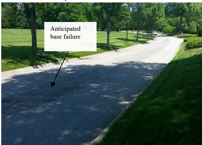
Photo #5: Southbound lane looking north
