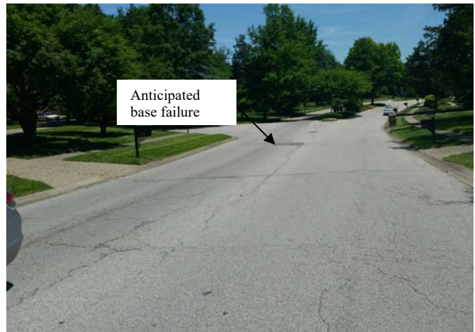
Photo #10: 2 way roadway section looking northeast just shy of northern median
