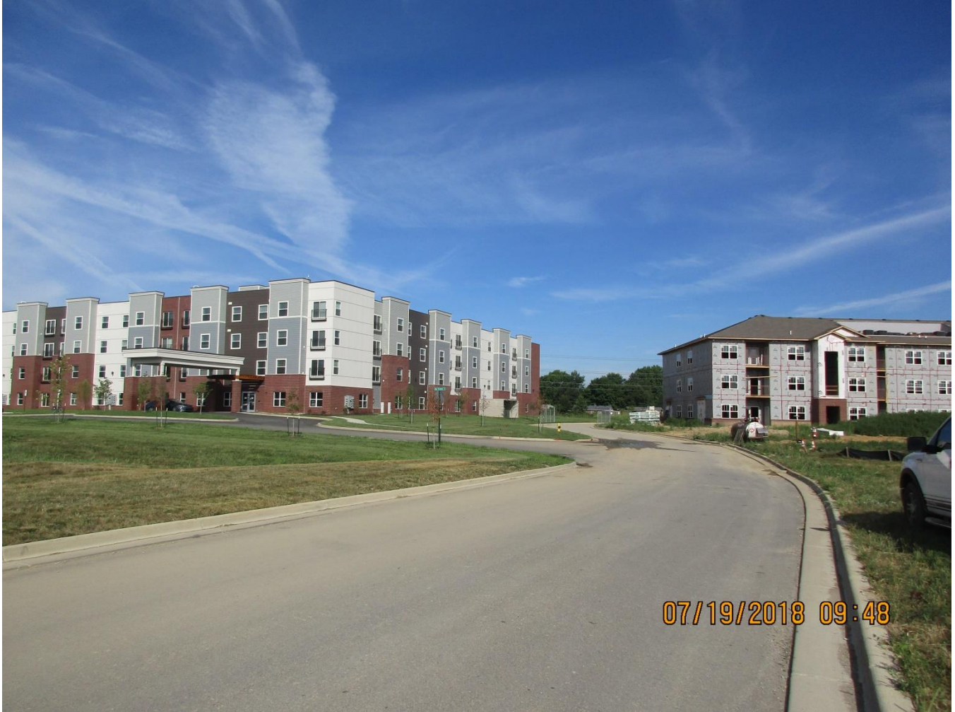
The interior of the site under construction.
