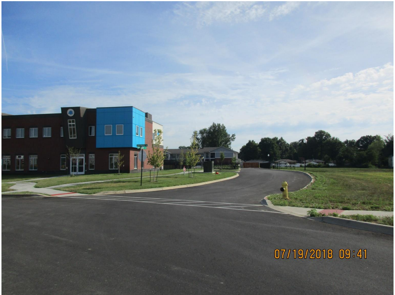
The site currently under development.
