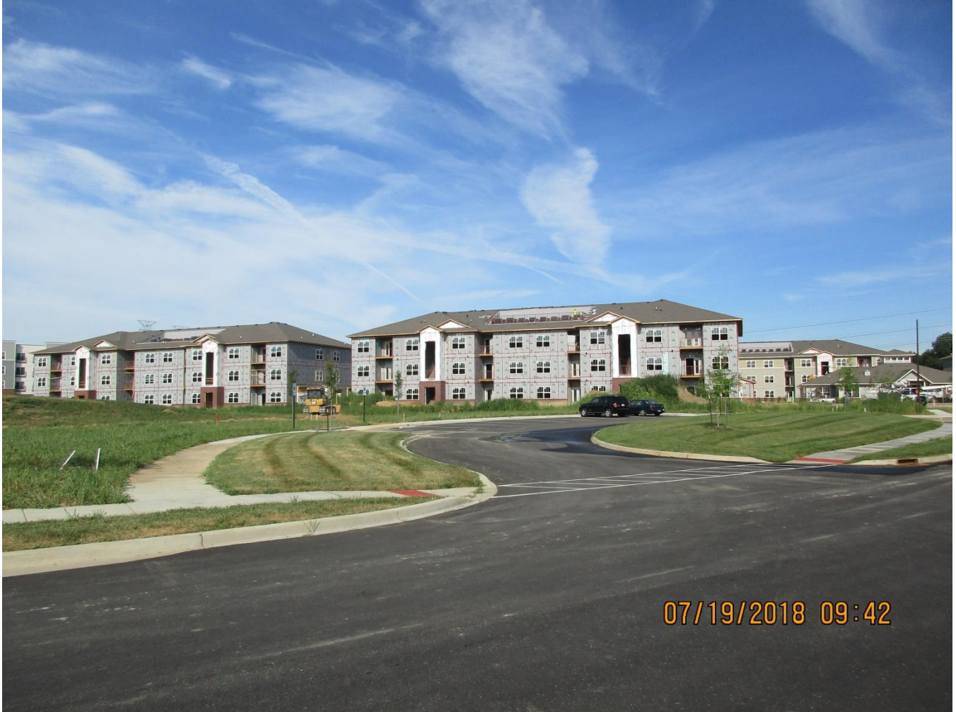
The interior of the subject property under construction.
