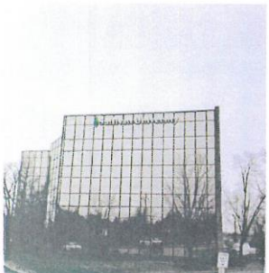
REMOVE THESE CHANNEL LETTER FROM LOCATION AT 207 Grandview Dr. Fort Mitchell, KY
