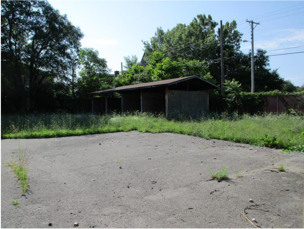
Taken from 22 nd Street sidewalk looking SE into the rear of site at existing rear building
