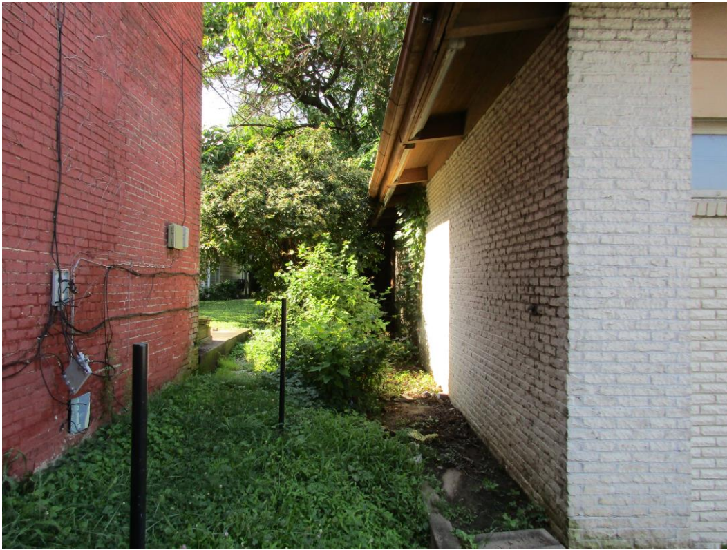
Close up of existing distance between buildings
