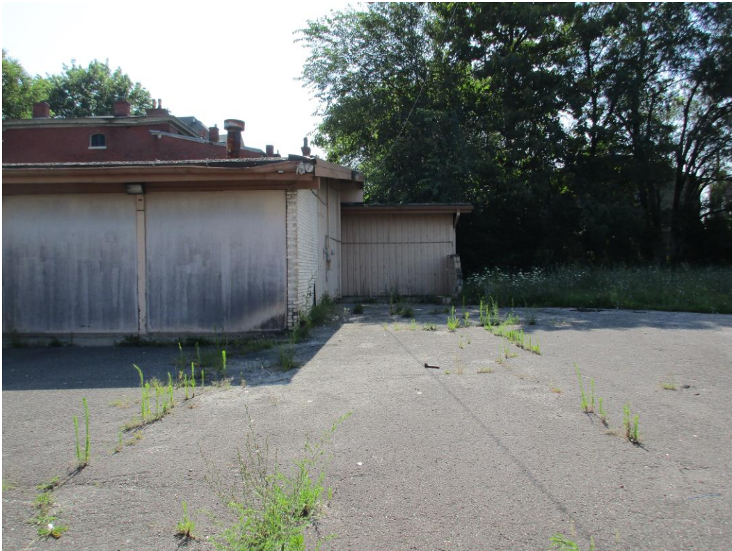
Taken from interior of site looking N at the existing pavement and rear of front building
