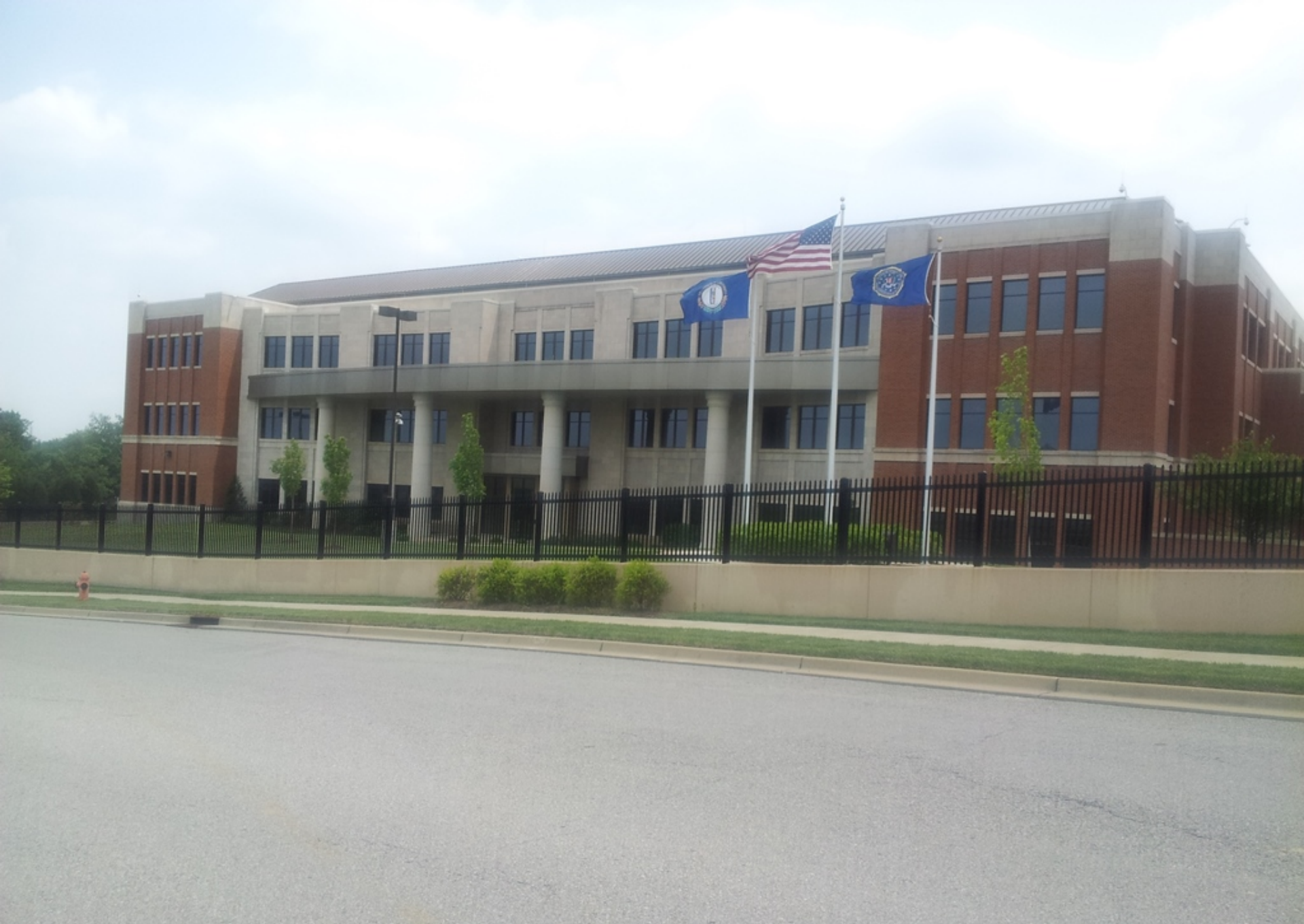
View of the FBI Building across from the site.
