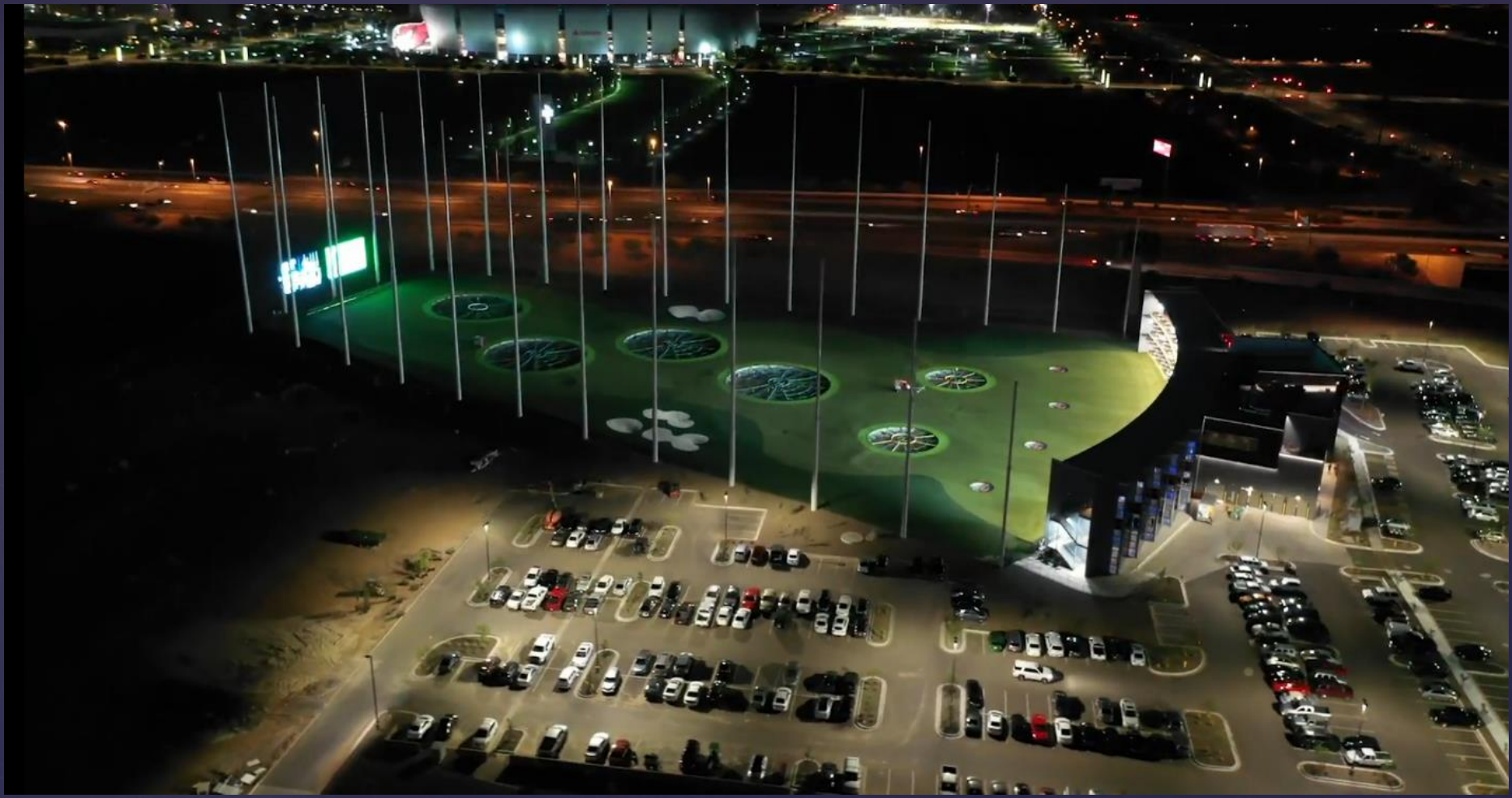
Glendale, AZ New lighting system
