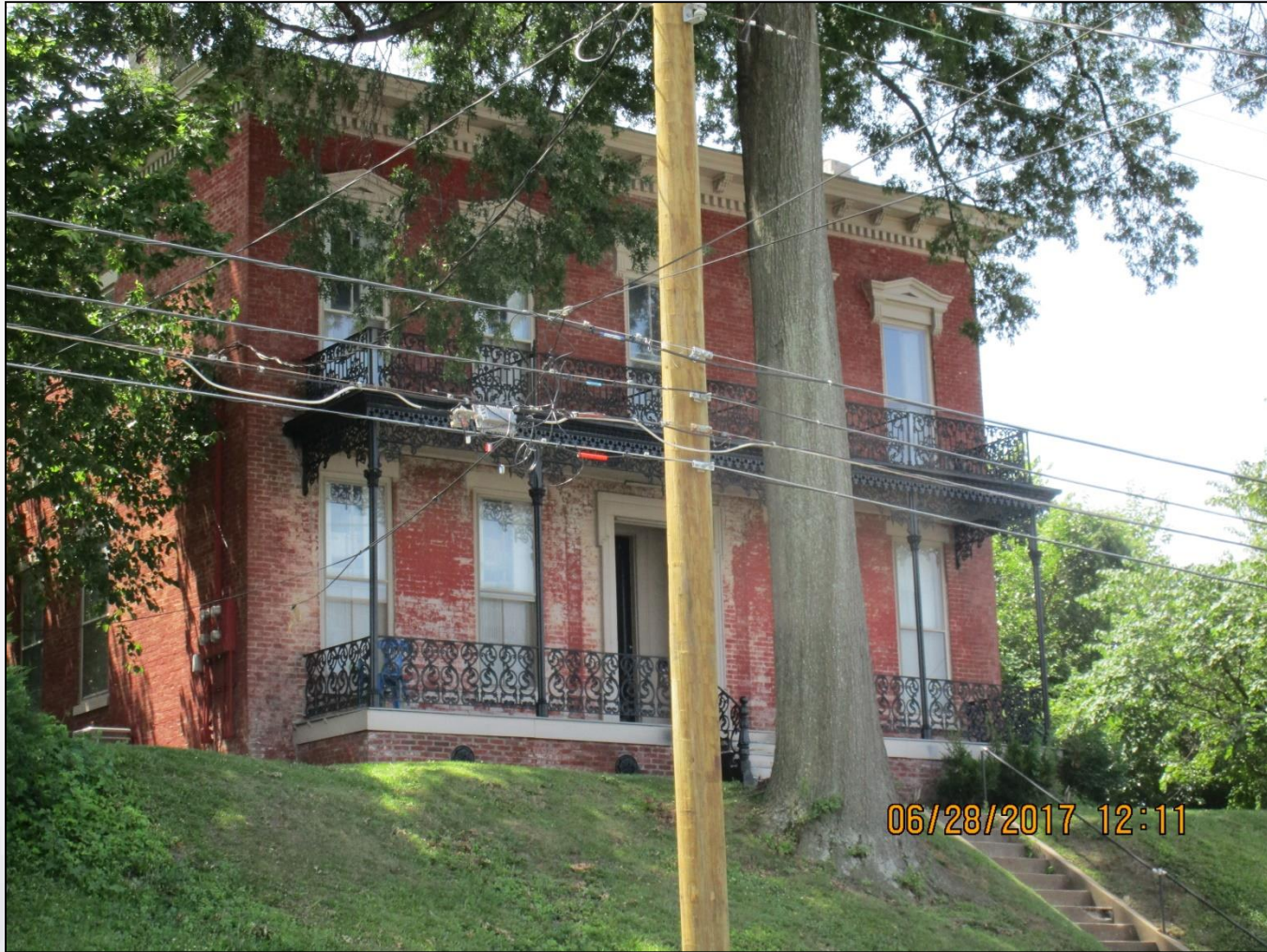
The multi-family residence to the west.
