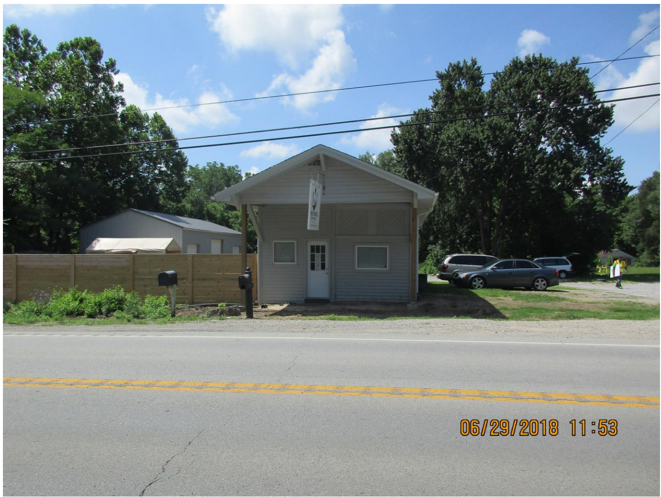
1. Front of property
