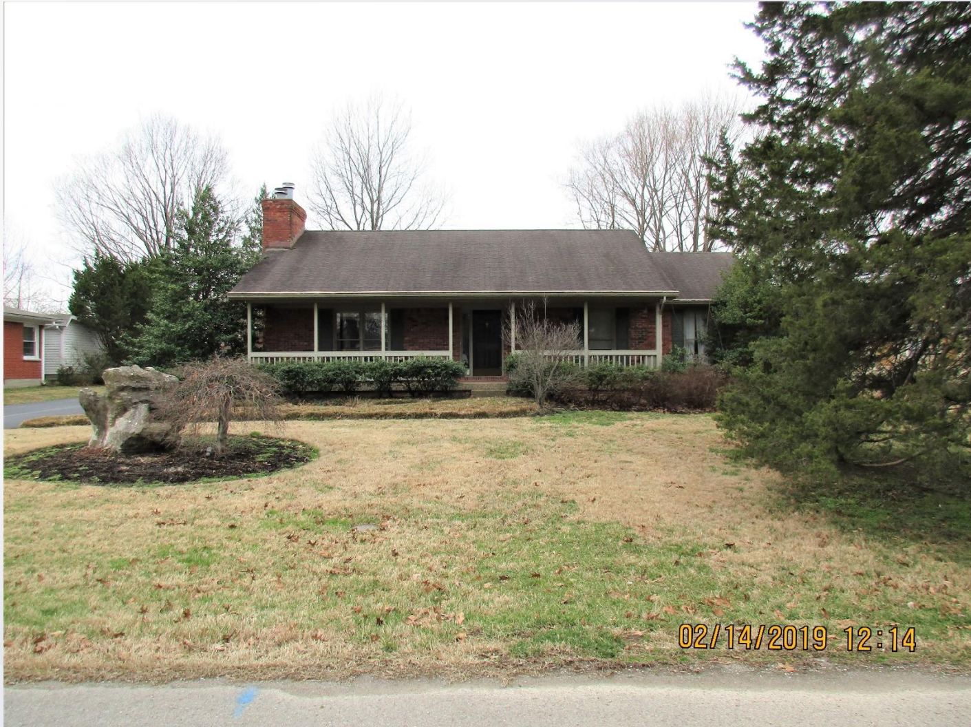
Adjoining to South
