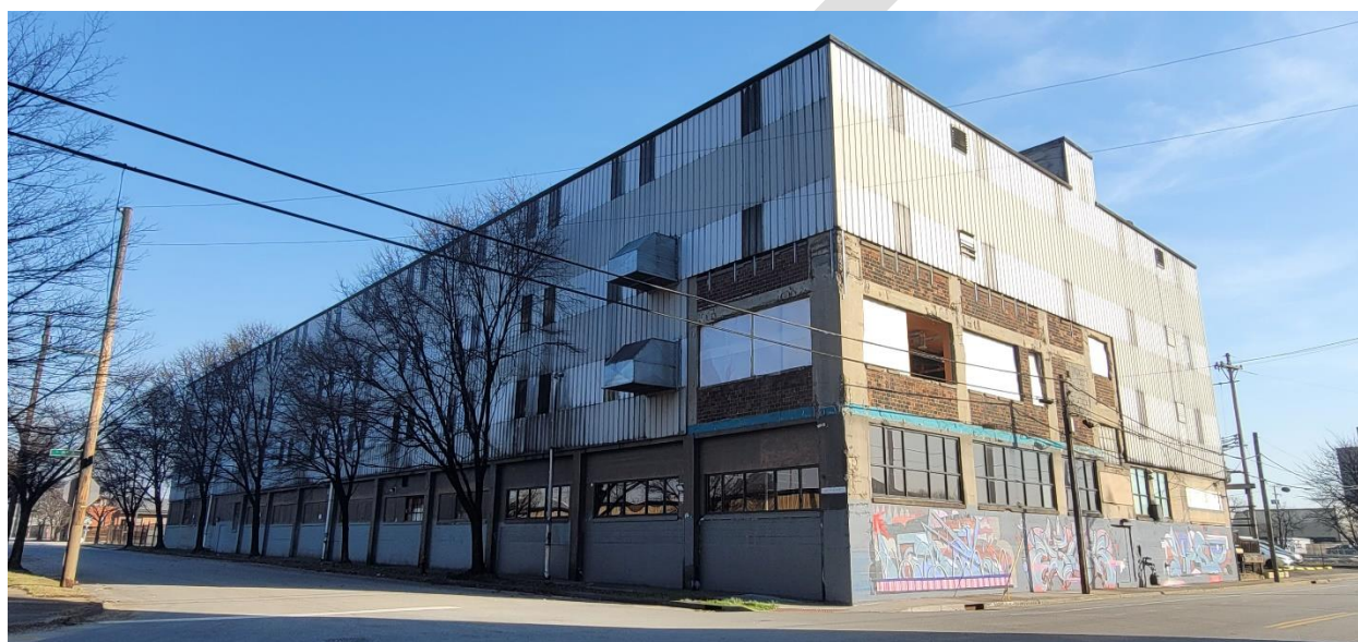
North and west facades after exploratory removal of metal panels began. March 2023. (C. Manzo)
