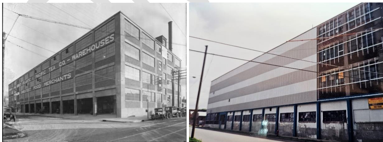
(Left) 1928 construction photo; (Right) 1996 installation of non-historic metal panels
