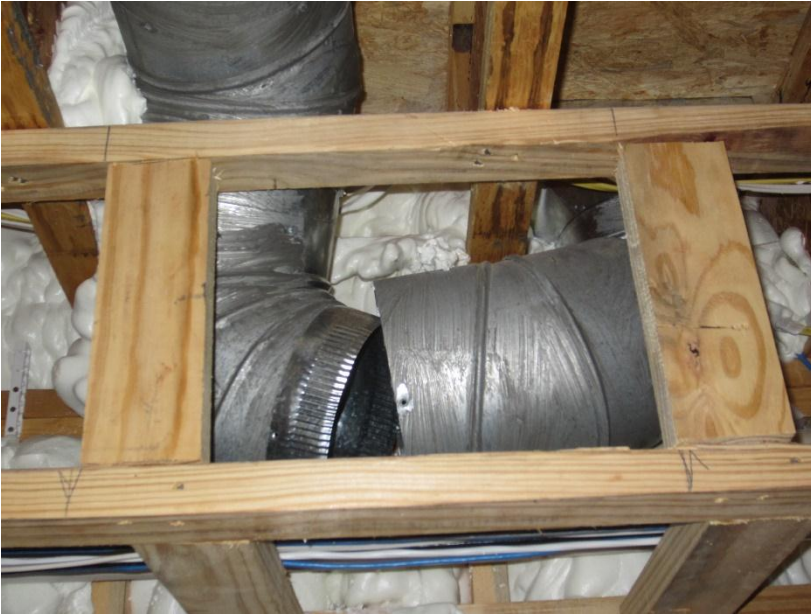
Disconnected Duct
