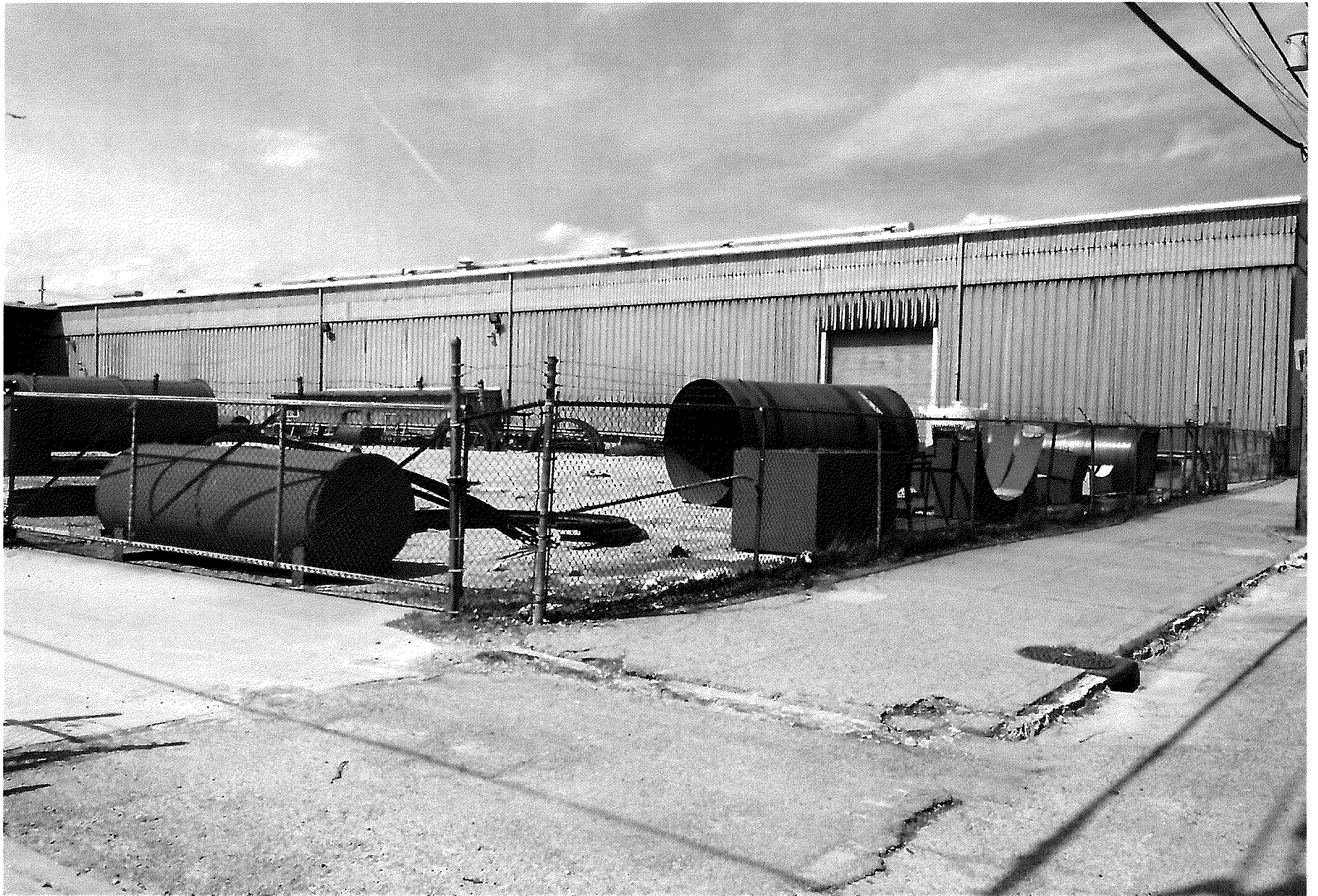
Service Welding Site north of Billy Goat Strut
