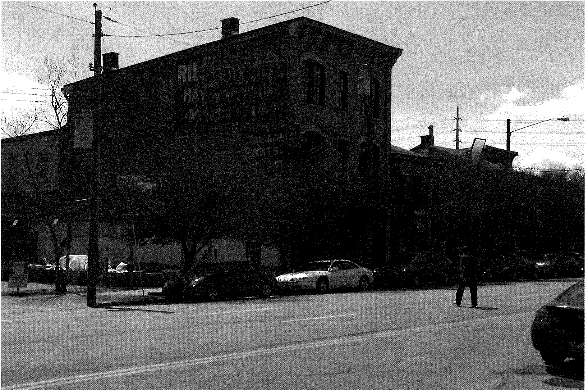
View south across Market Street
