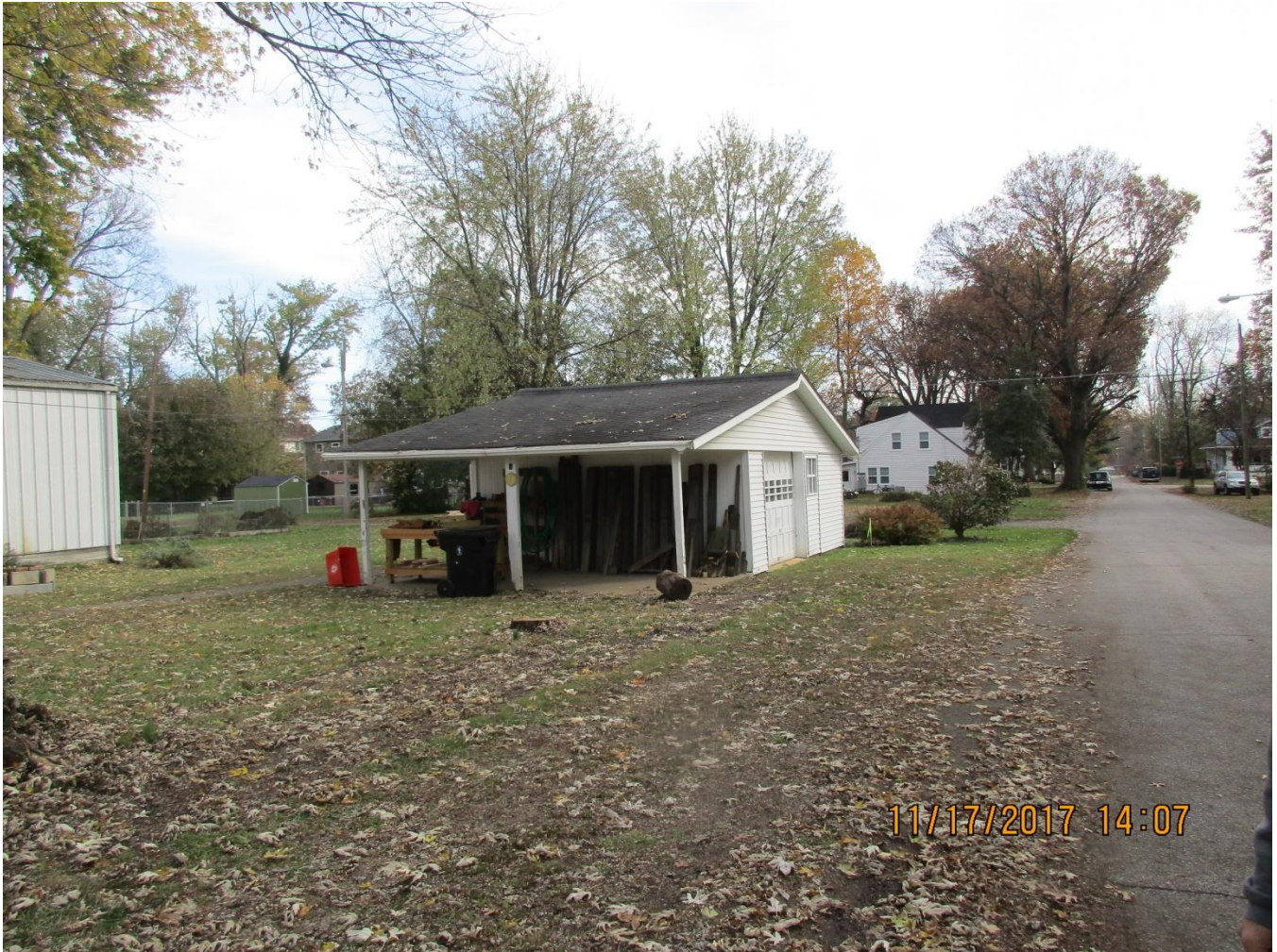
The existing garage to be removed.
