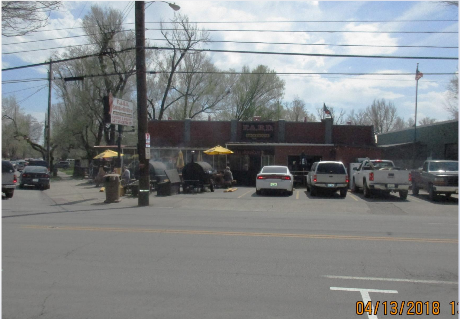
Adjoining Property to East
