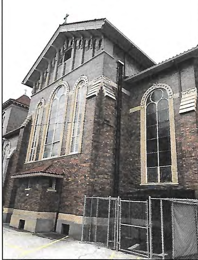
Figure 5. North elevation of Building 1, looking southeast.
