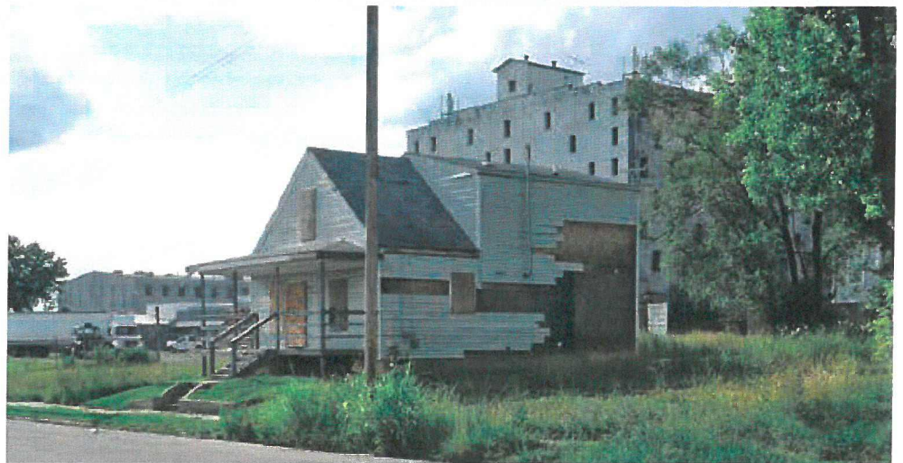
A flood-damaged home on West Market Street awaits demolition.
