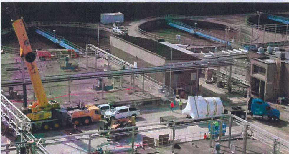
The new oxygen generation equipment is delivered to the site.
