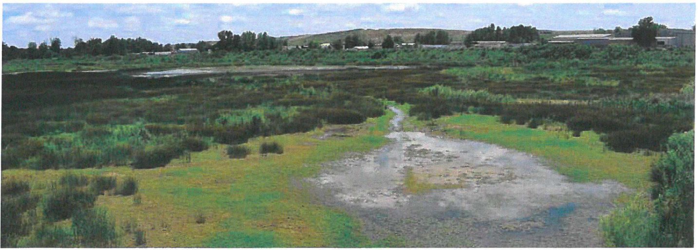
Above: The 64.9 acre Melco Basin can capture and store nearly 489,000,000 gallons of rainwater, providing flood protection to the surrounding area.
