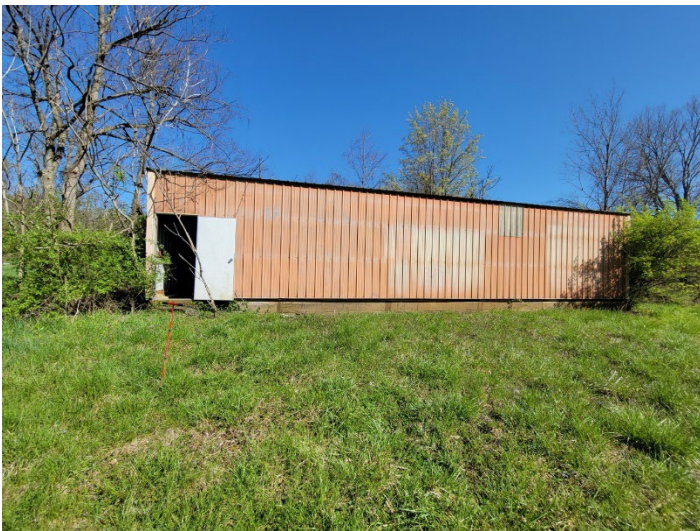
Photo 57 – View of remnant shed
