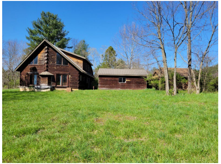
Photo 56 – View of remnant house
