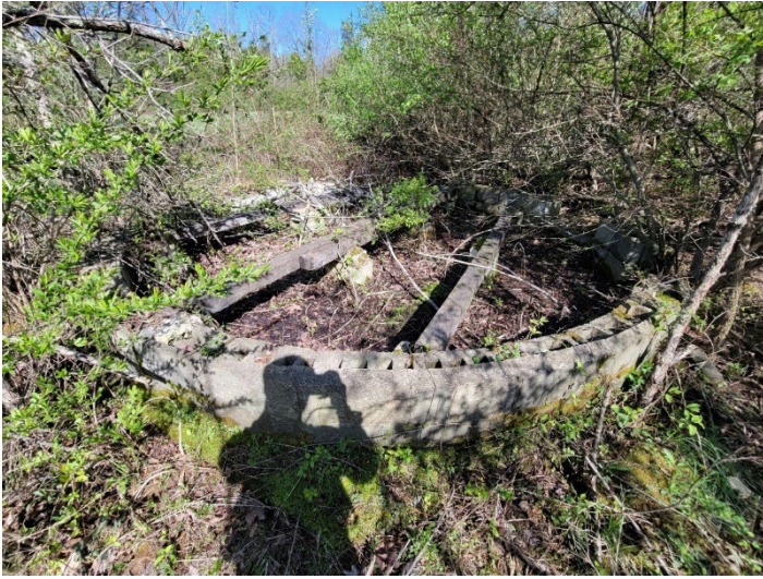
Photo 55 – View of remnant foundation
