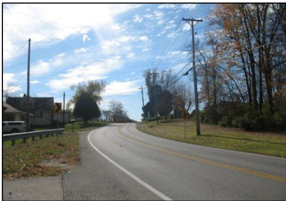
Manslick Road at Holly Park Drive looking to the south at one of several deficient vertical curves.
