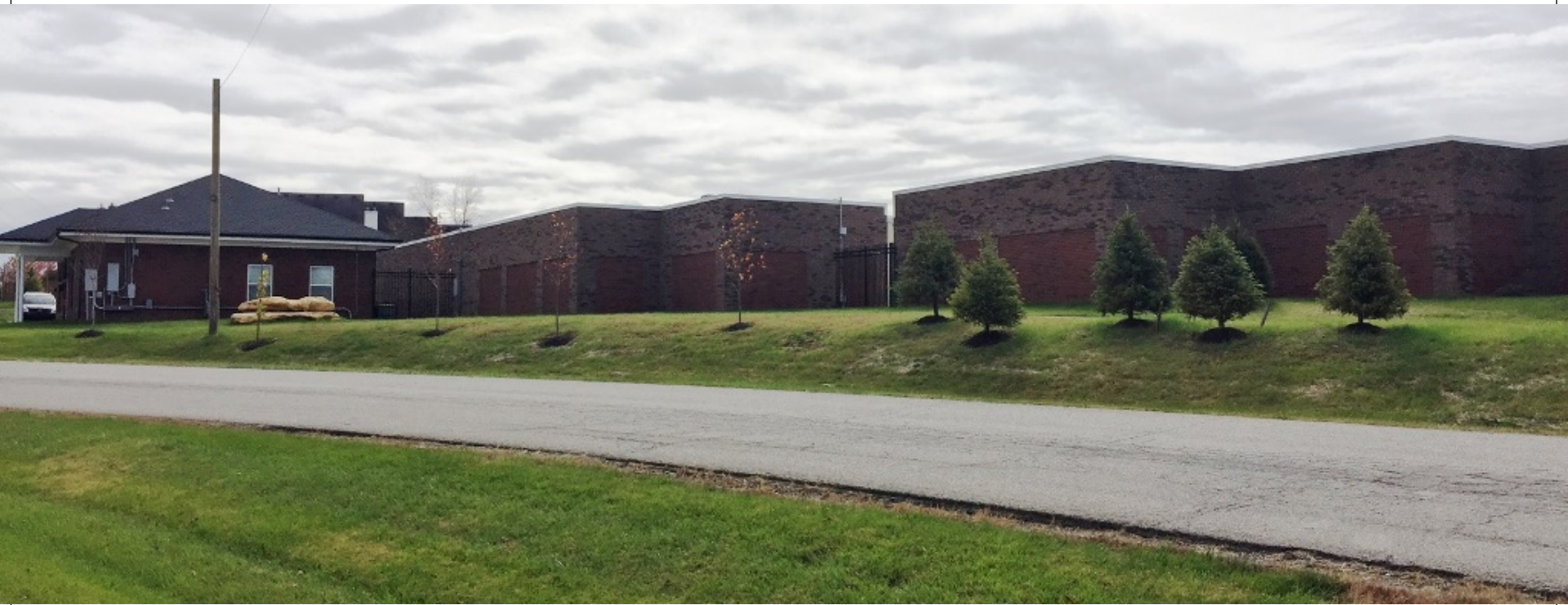
Representative photograph of the mini-warehouse facility
