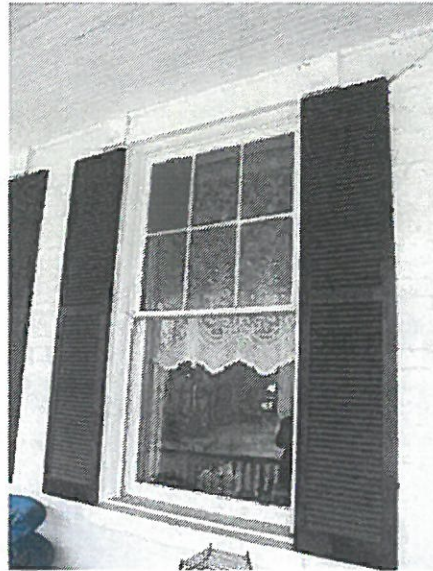
(Above-left) This is a photo of the two windows at the right side of the façade, sheltered by the front porch. (Above-right) This is a detail photo of one of the 6/1 wooden d.h. façade windows sheltered by the front porch. (Below-left) This is a detail photo of the shed roof front porch. (Below-right) This is a detail looking NW out from the front porch.
