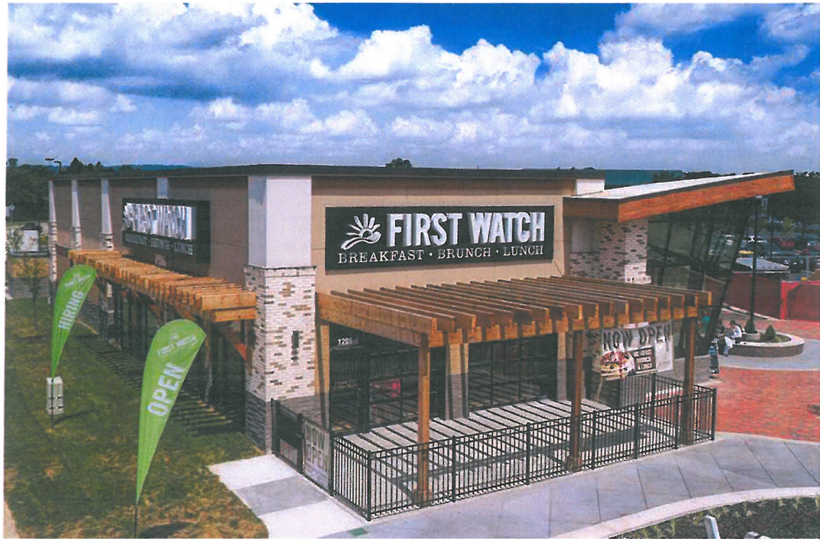
Photo Above: First Watch - Clarksville, built example of this design prototype.
