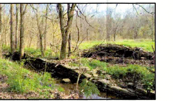
24 VIEW TO SOUTH AT DRAINAGE WAY
