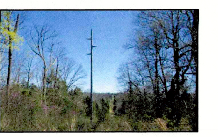
16 EDGE OF OPEN FIELD LOOKING DOWN ESMT
