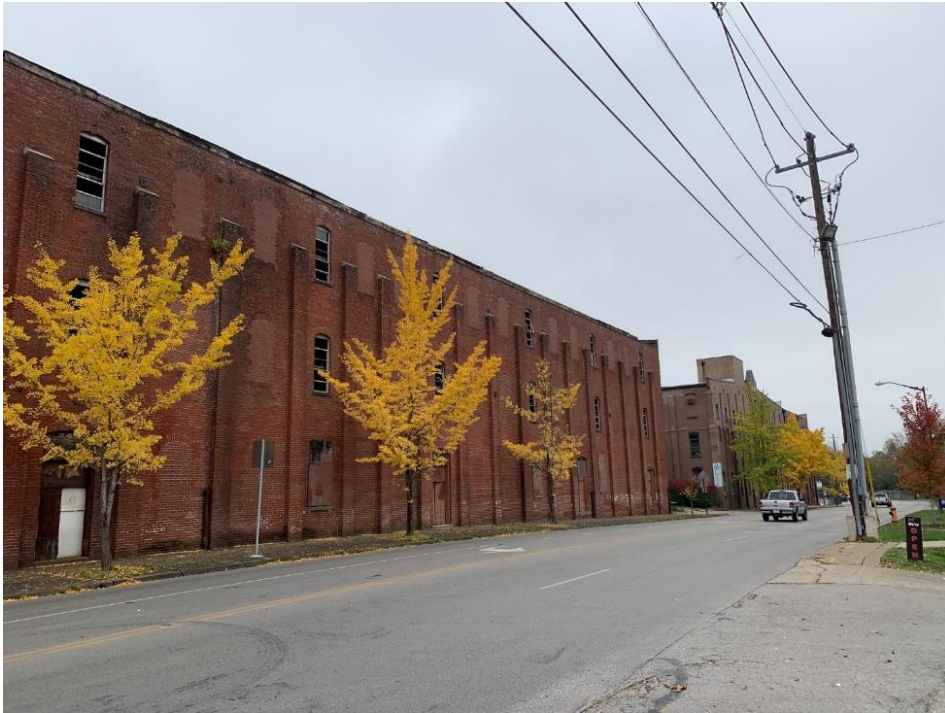
North Elevation (Staff Photo October 2020)
