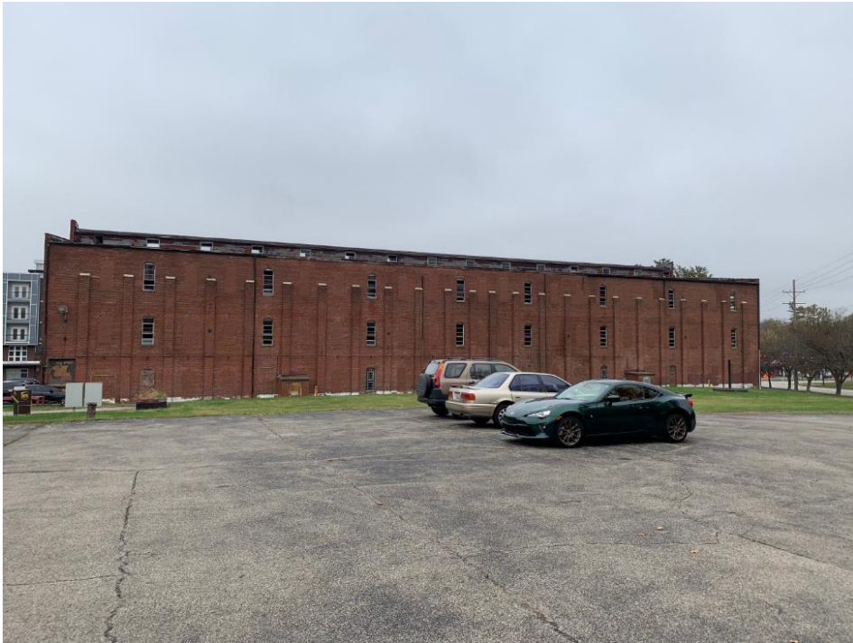
South Elevation (Staff Photo October 2020)
