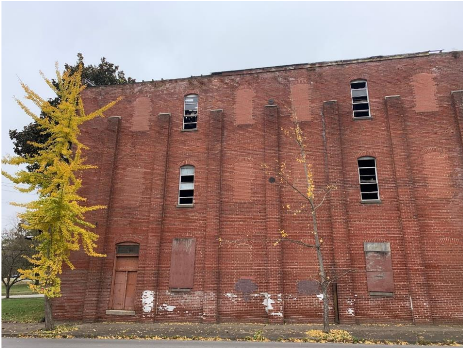
North Elevation (Staff Photo October 2020)
