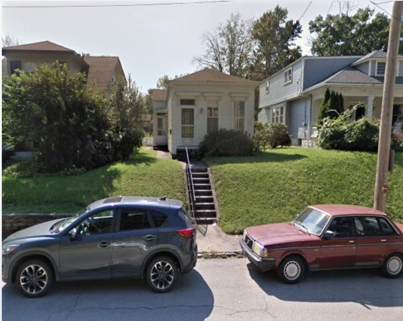
Adjacent to East
