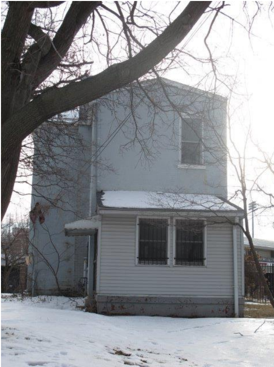
Photo 4: West (rear) elevation
