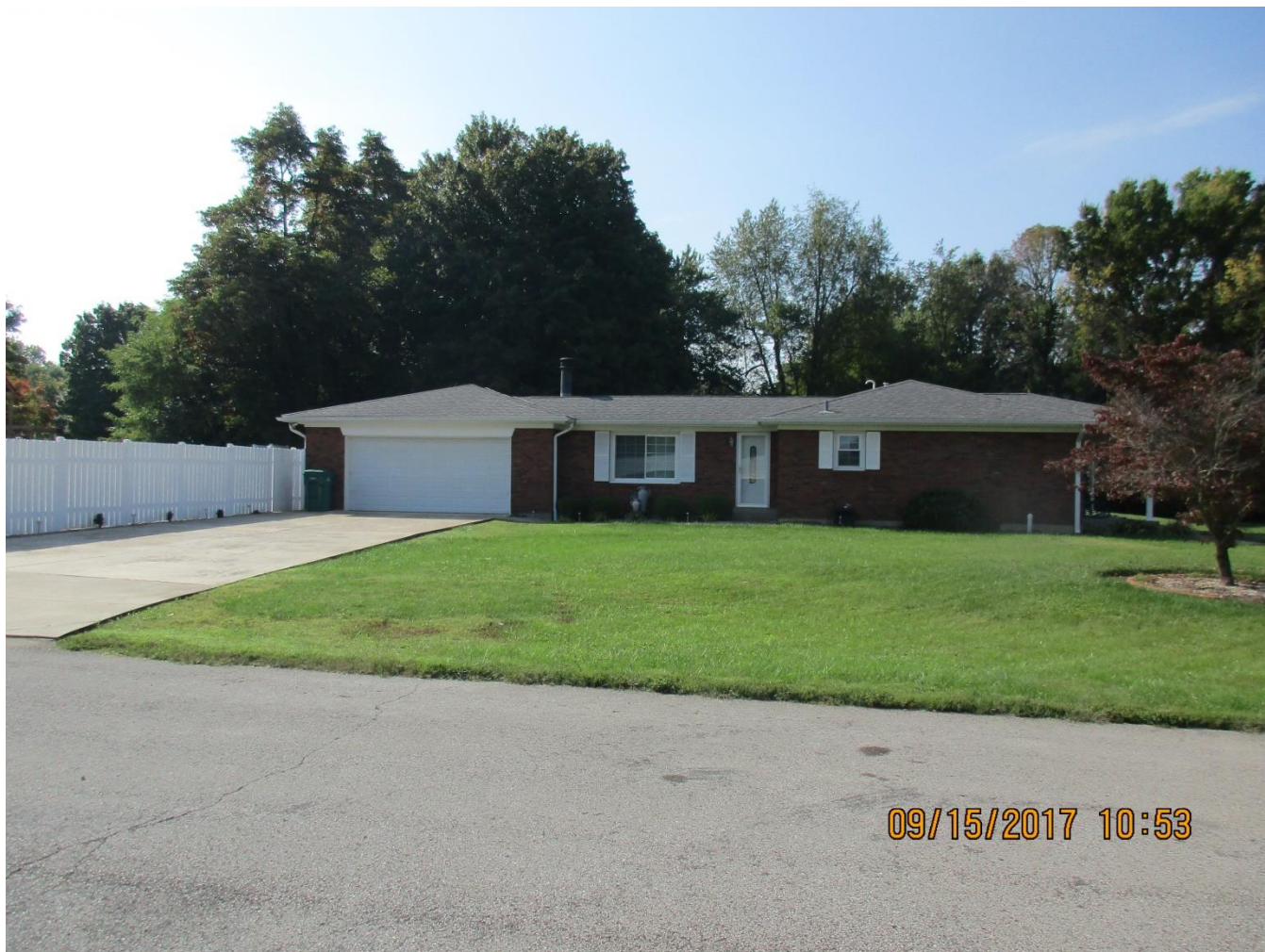
The side of the subject property, where the addition is proposed to extend into the yard.
